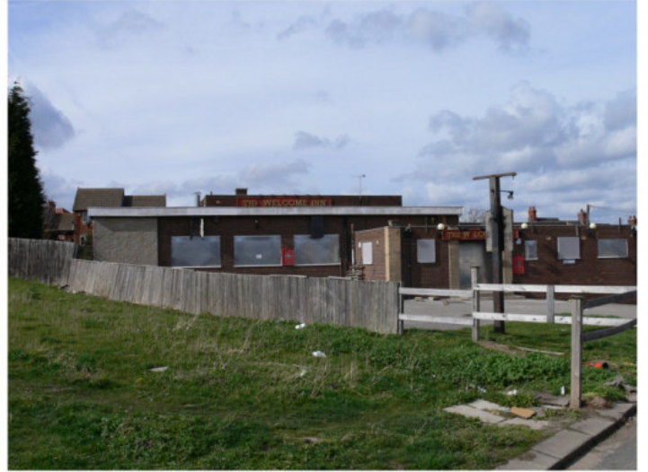
EXISTING PUBLIC HOUSE TO NORTHERN BOUNDARY
