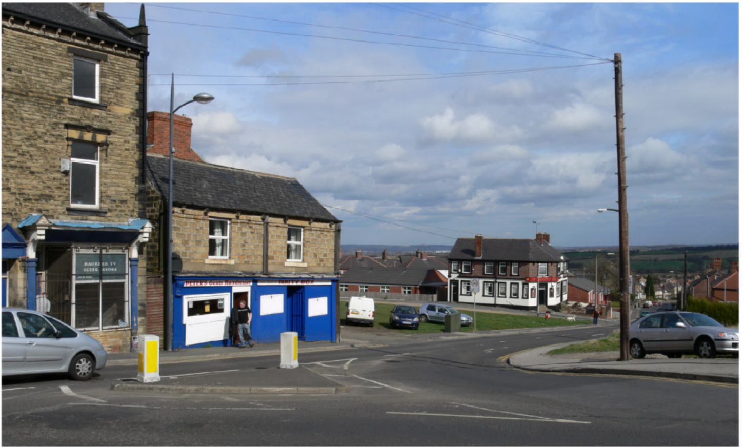
HIGH STREET - EXISTING VIEW FROM THE WEST
