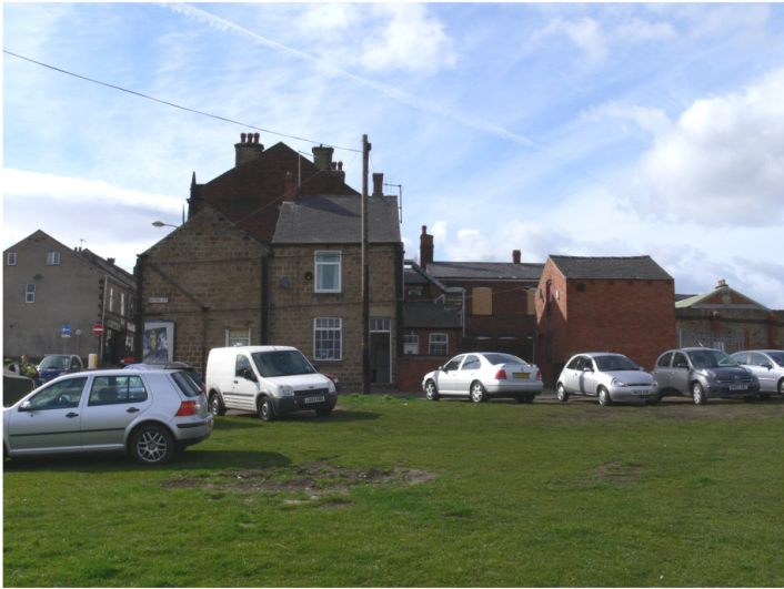
VIEW TOWARDS BETHEL ST
