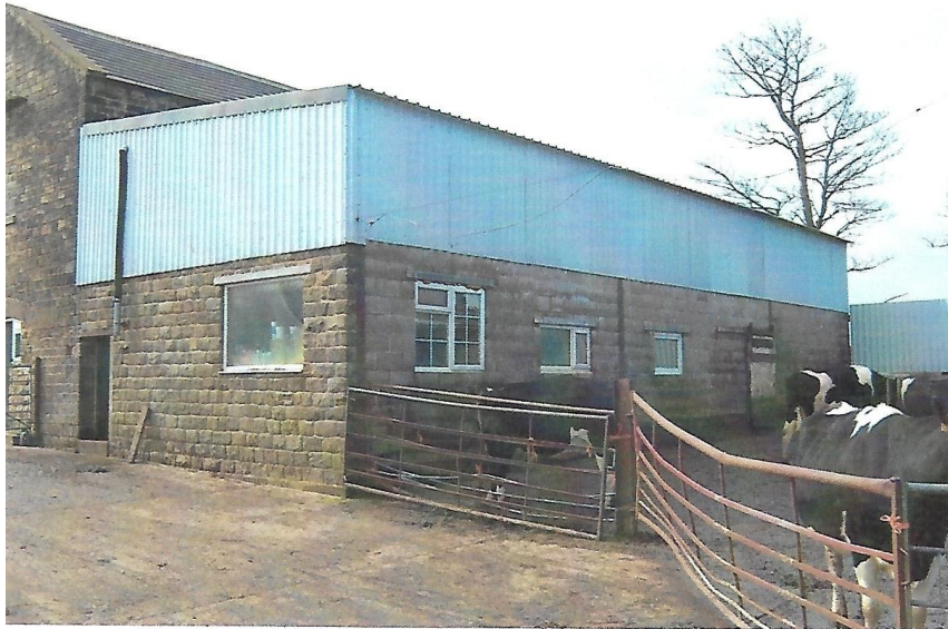
Original lean to, North Elevation
