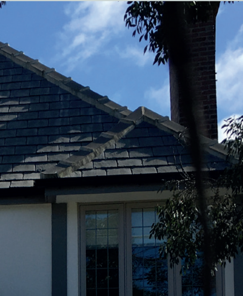
Greys Artstone GRC Slate (Glassfibre Reinforced Concrete)
