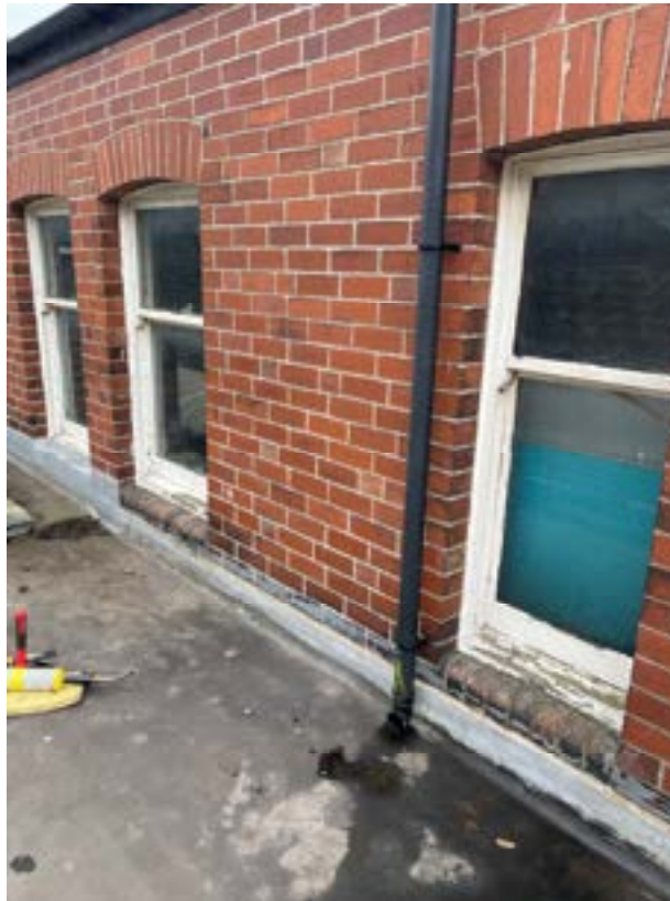
Timber Framed Sash Windows to be Replaced
