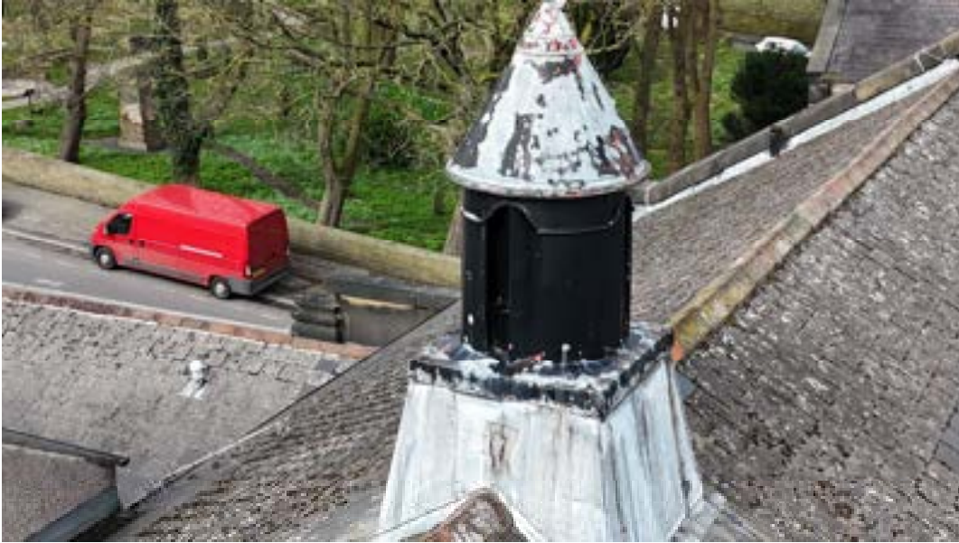
Typical Roof Cowl to be Removed
