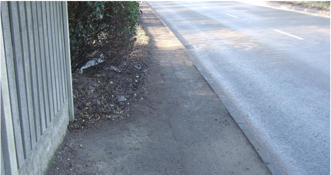
Figure 3 Shaw Lane footway narrowing to 700mm wide west of the proposed toucan crossing
