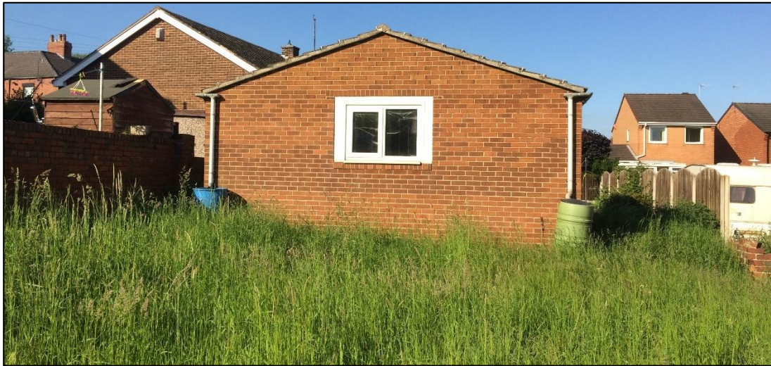
Plate 6. Garage, dwelling with improved grassland in foreground.
