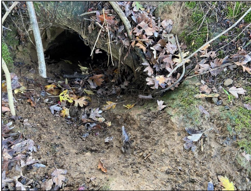
Photograph 2 showing one of the larger holes within group
