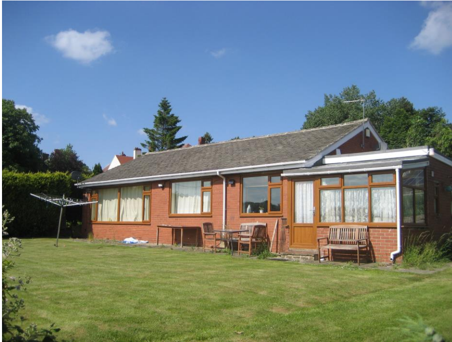
View of western elevation
