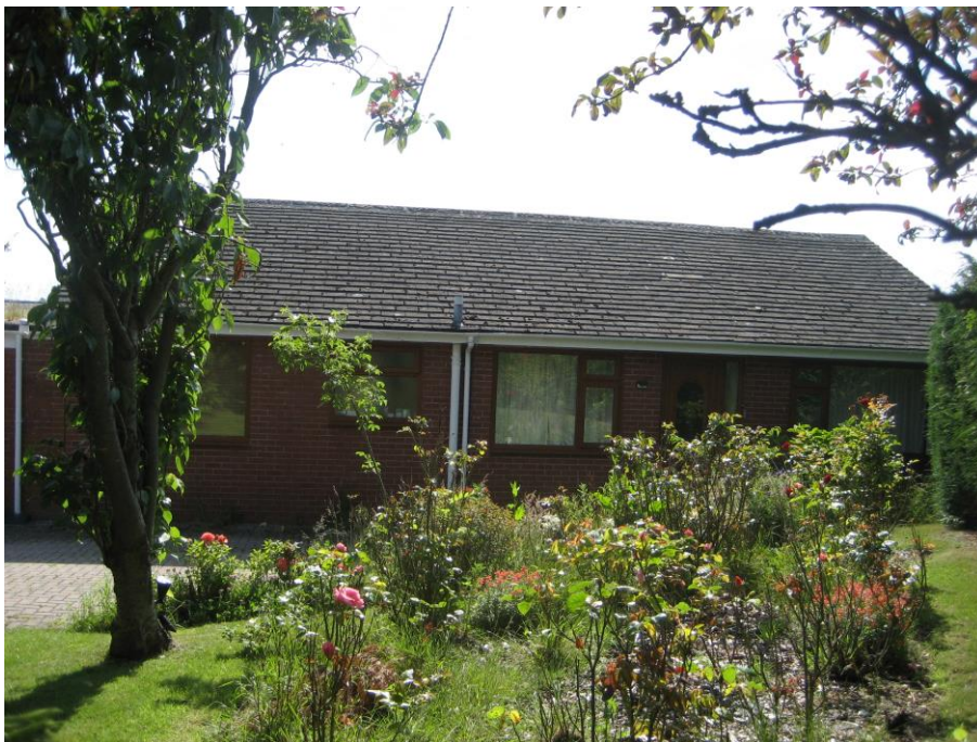
View of eastern elevation.
