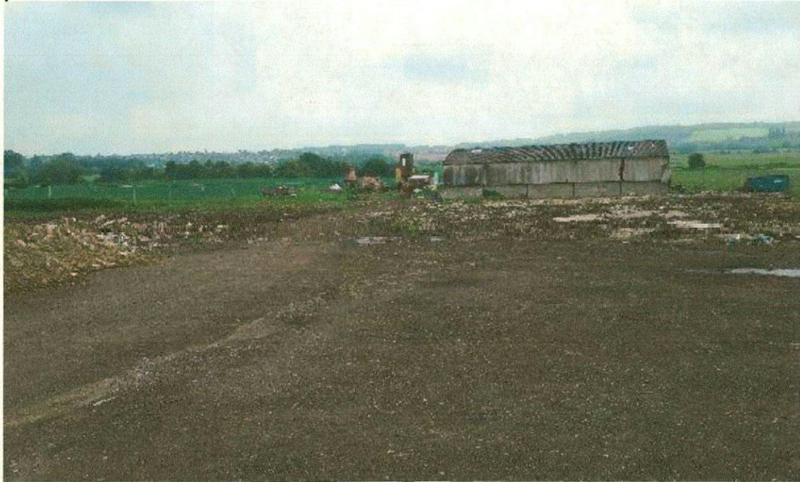
Photo 1. Looking north across the site towards the agricultural shed with negligible potential for bats
