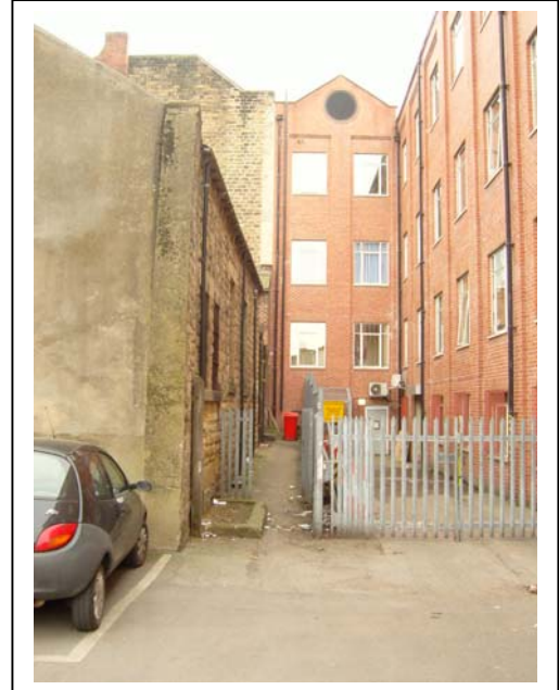
View of 45 Market Street from the rear of 39-43 Market Street
