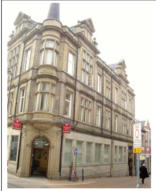
Front View 45 Market Street
