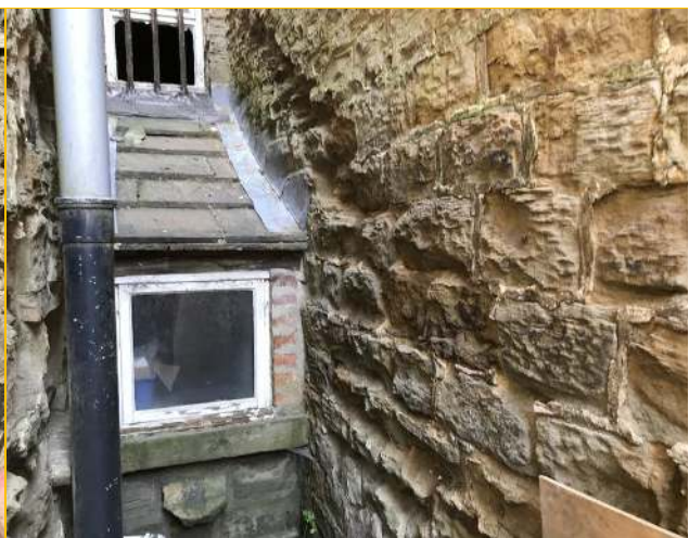
Photograph - 38 - Weathering
