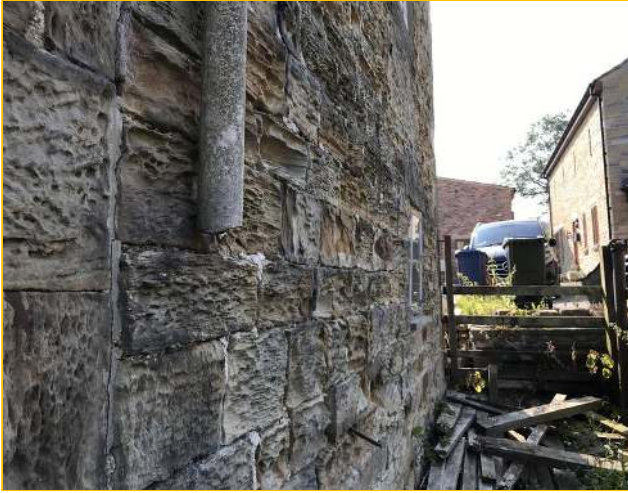
Photograph - 17 - Right extension
