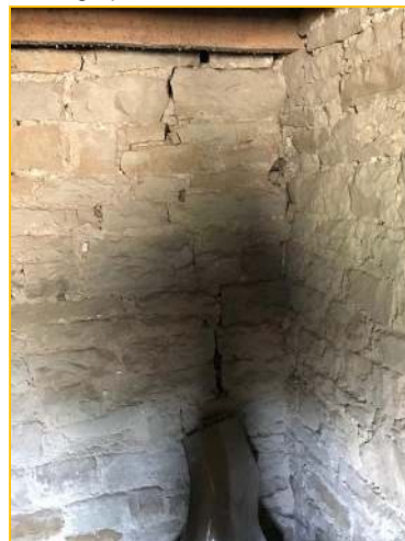
Photograph - 67 - Right extension
