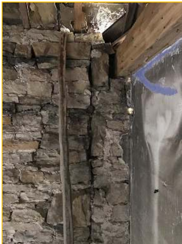
Photograph - 61 - Right hand extension
