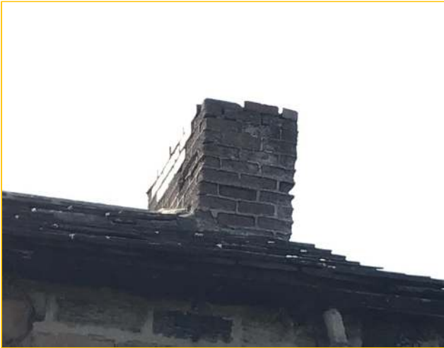
Photograph - 42 - Brickwork stack
