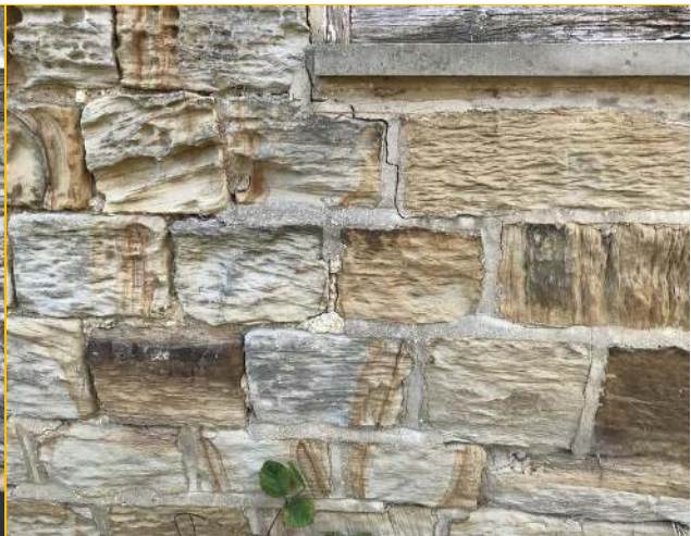
Photograph - 20 - Right extension
