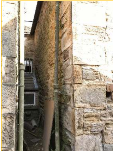
Photograph - 13 - Left extension right wall
