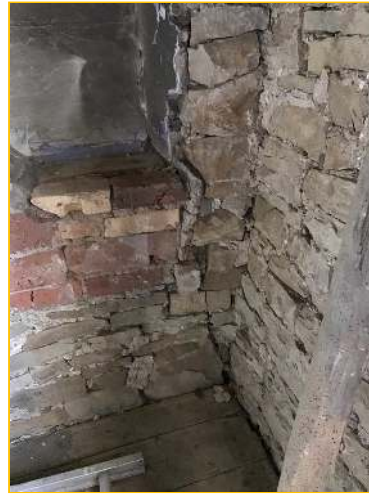
Photograph - 63 - Right hand extension
