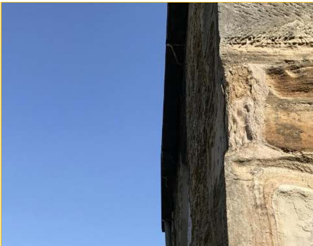
Photograph - 9 - Rear eaves line
