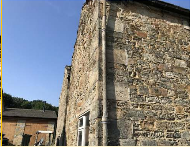
Photograph - 24 - Left extension
