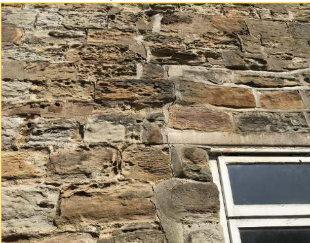
Photograph - 27 - Left extension
