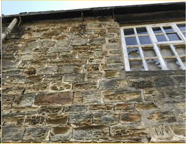
Photograph - 18 - Right extension
