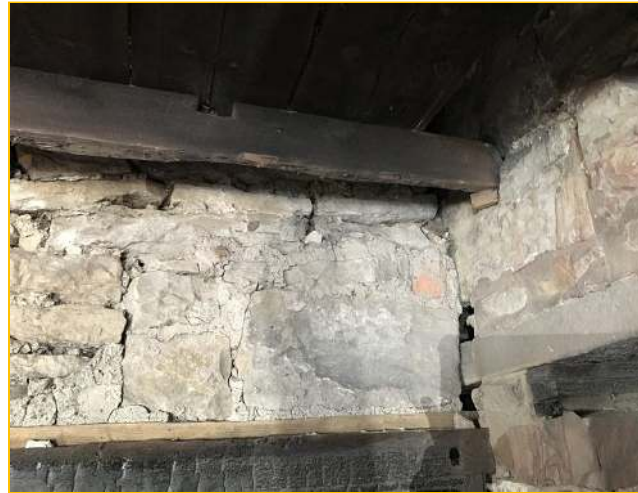
Photograph - 72 - Reflected fracture
