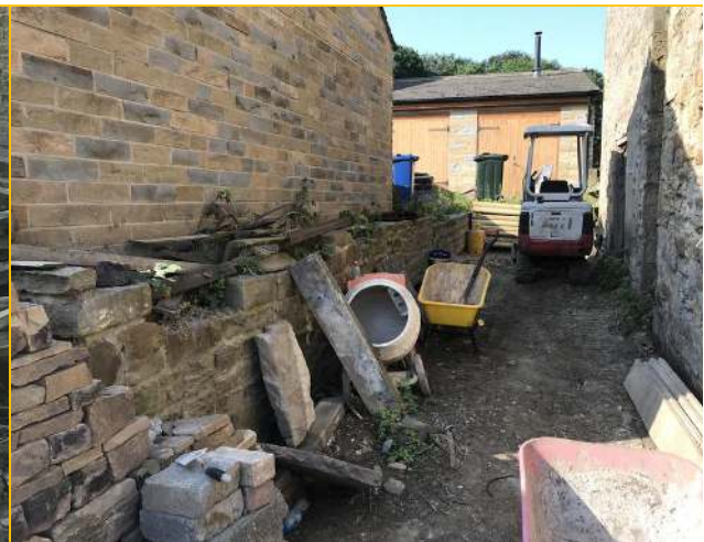
Photograph - 4 - Rear boundary walls
