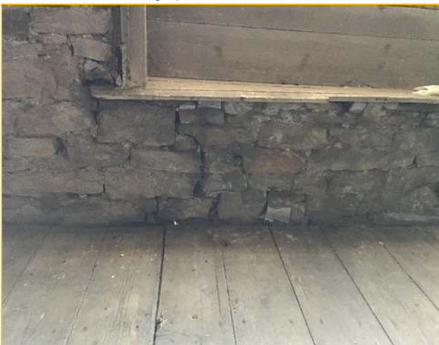
Photograph - 70 - Right extension
