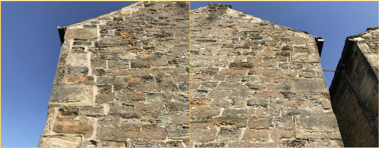
Photograph - 32 - Right extension
