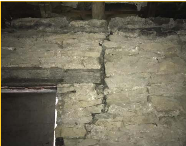
Photograph - 68 - Left extension
