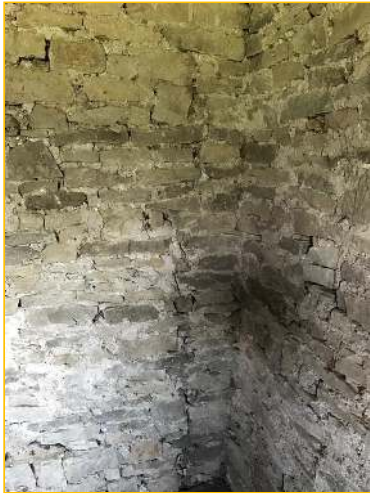
Photograph - 62 - Right hand extension
