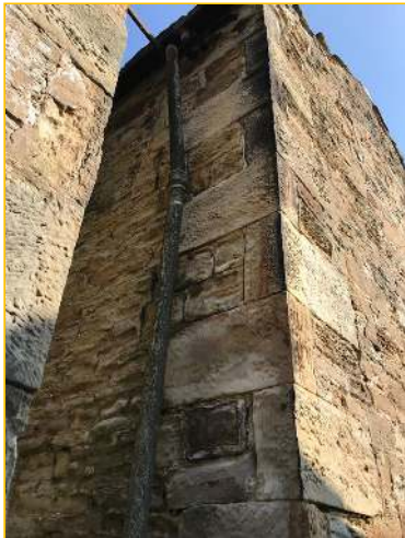
Photograph - 34 - Left extension
