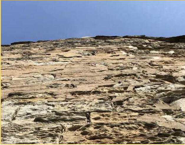
Photograph - 23 - Left extension
