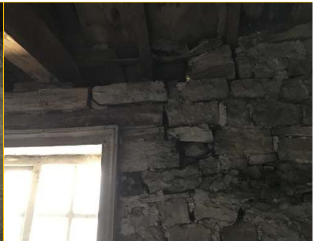
Photograph - 69 - Right extension
