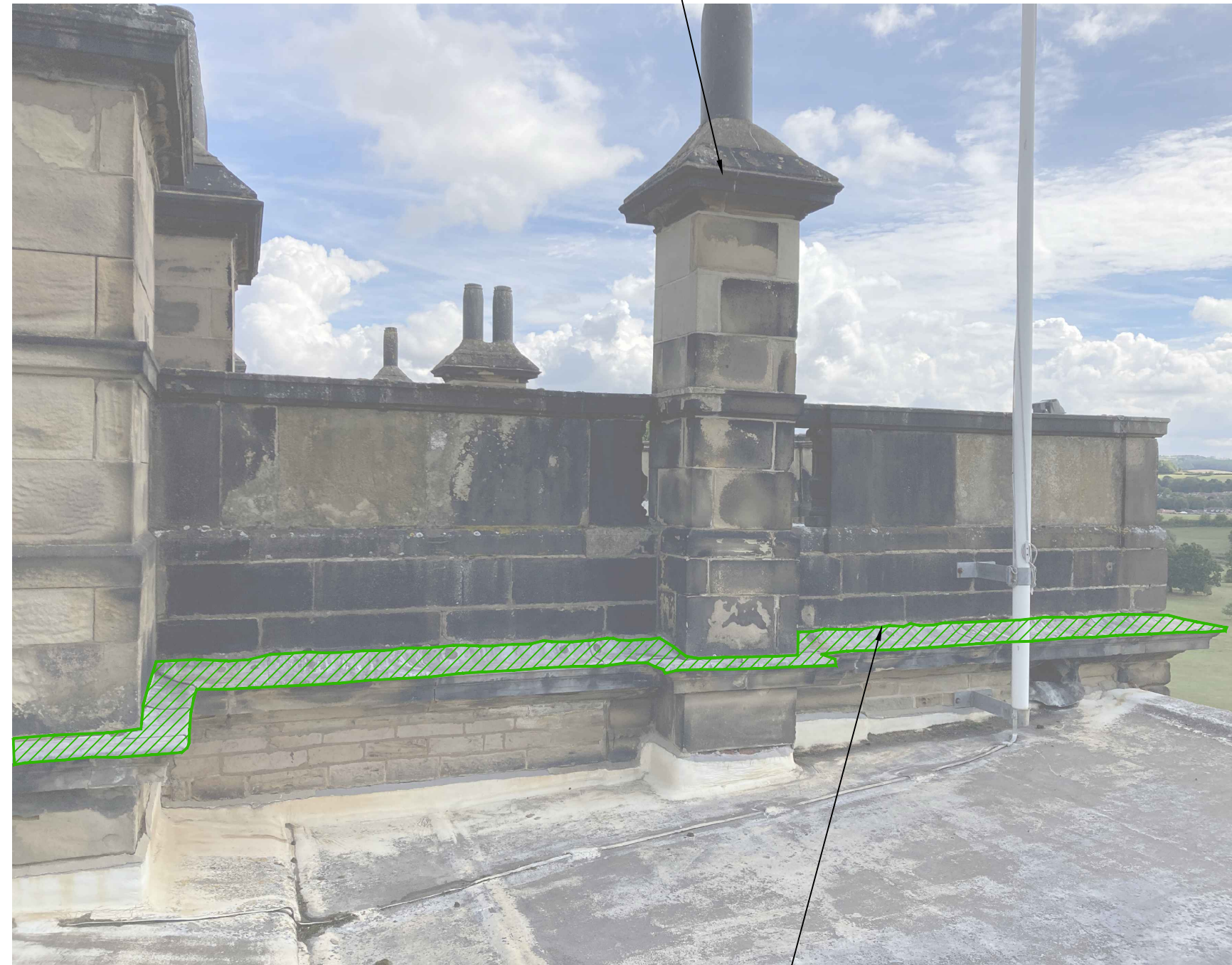
Photograph 5 Renew lead flashing with Code 5 lead, finished with lead mastic
