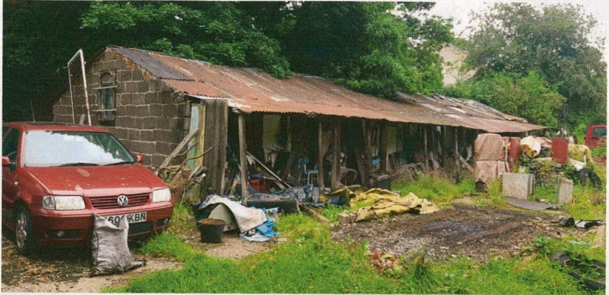
Photograph from the South West Showing the Appearance of the Existing Building.
