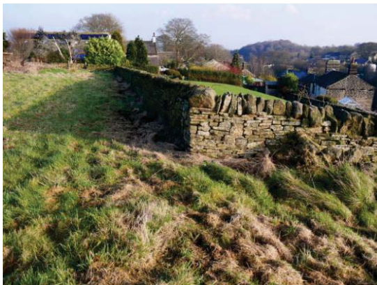
Plate 12: Modern dry stone boundary wall of White House Farm garden located within the southeast corner of the new development site
