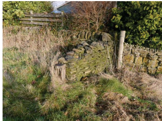
Plate 3: Remains of a dry stone wall abutting the eastern boundary wall
