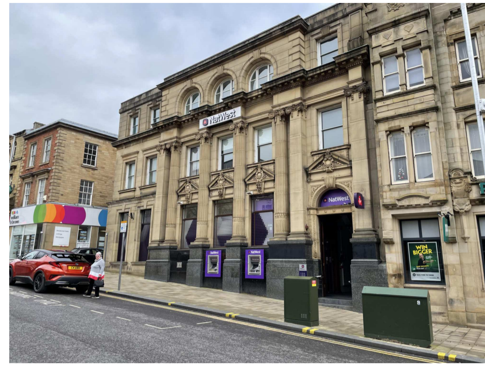
1. Main View of Market Hill Rd
