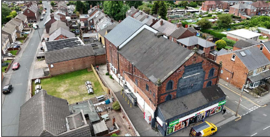
Plate 2. The building viewed from the northeast
