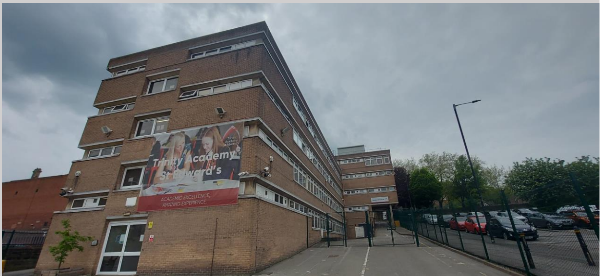
Photograph 7: Image taken facing west to the rear of Trinity Academy including hardstanding ground and Paladin fencing.
