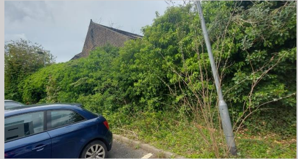
Photograph 6: Image of stone wall located to the north of the site's boundary covered with Ivy. This wall is to be retained and unaffected by works.
