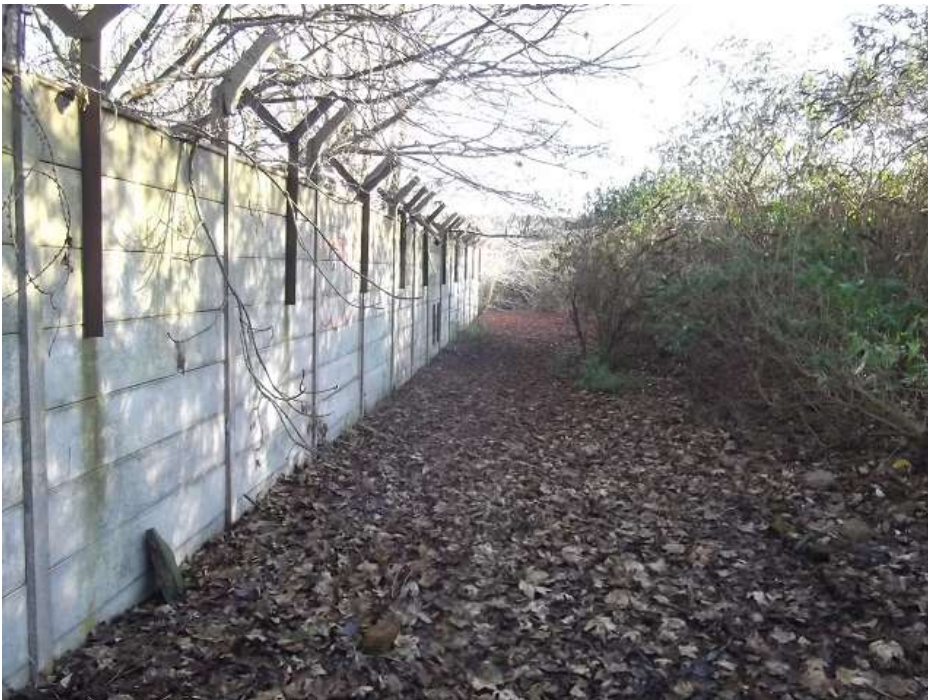
Plate 6. Looking east along the northern boundary concrete panel wall.
