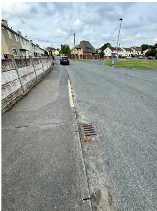
7 - Gully and patch work in footpath
