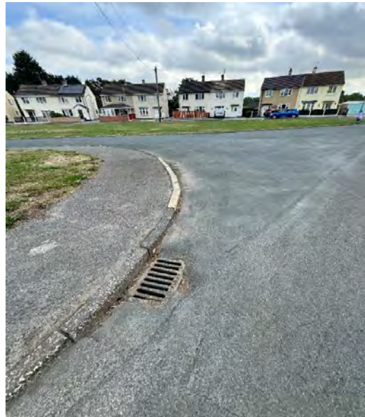
18 - Gully in good condition
