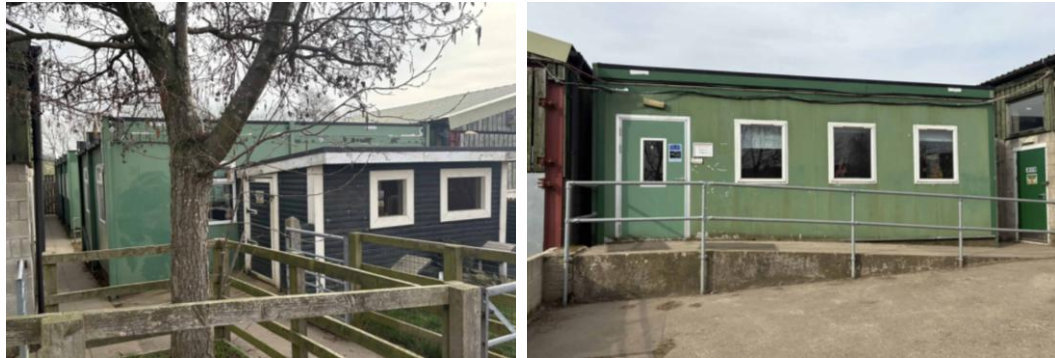
BUILDINGS REMOVED FROM SITE (PHOTO TAKEN – JULY 2026)
