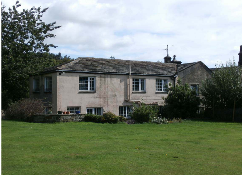
Figure 3 General view of the extension from the North West.
