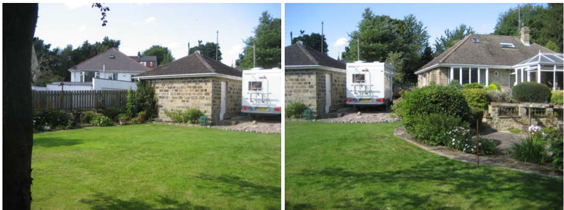
The site and the existing buildings viewed from the south.
