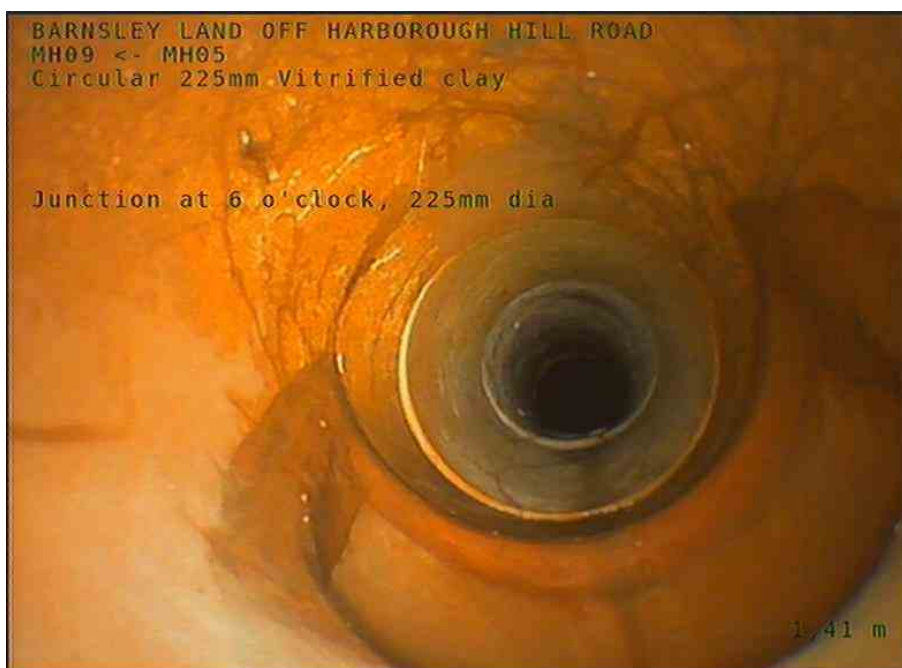
1, 00:00:23, 1.41 m Junction at 6 o'clock, 225mm dia, BACKDROP
