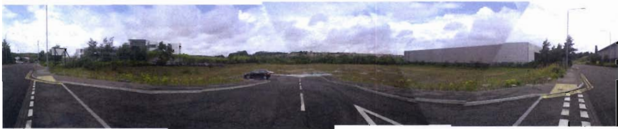
Panoramic view of site from Cortonwood Drive from the south-east
