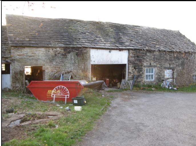
The barn (surveyed building) at Water Slack Farm.
