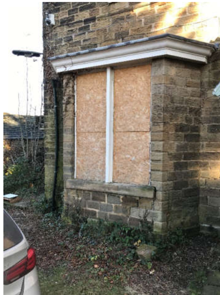
Fig 14. Bay window adj porch to west elev.
