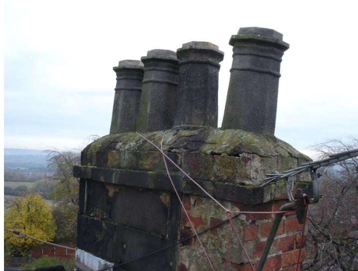
Fig 16. Close up view of main chimney stack in ashlar with brick addition.
