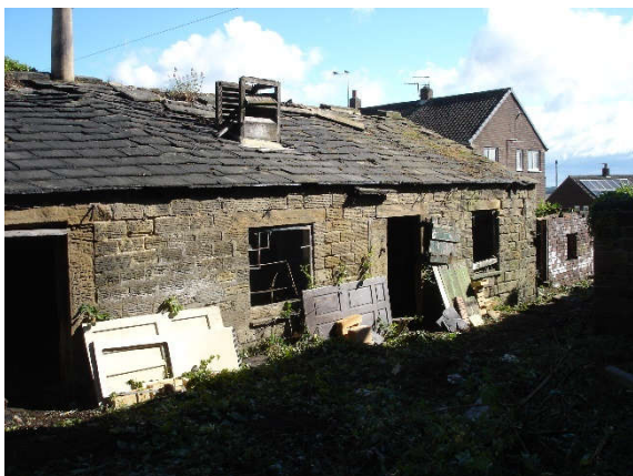
Fig 09. Stone Outbuilding to rear.
