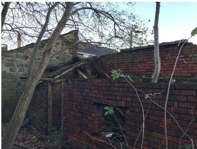
Fig 23. Lean-to brick Outbuilding.
