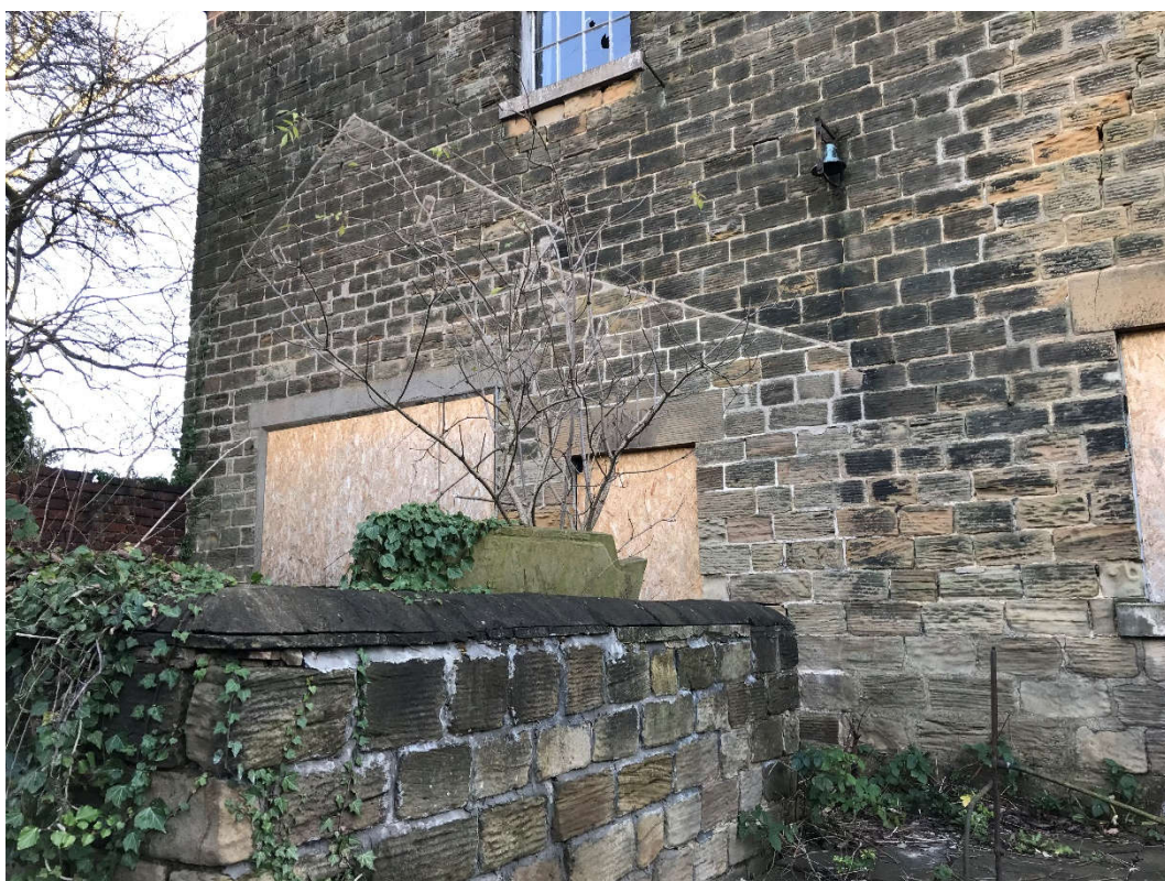
Fig 21. North East rear corner of house showing outline of former building now removed and dwarf wall around terrace, possibly original external wall of former building.
