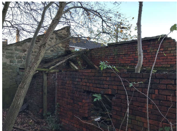
Fig 10. Brick Outbuilding to rear.
