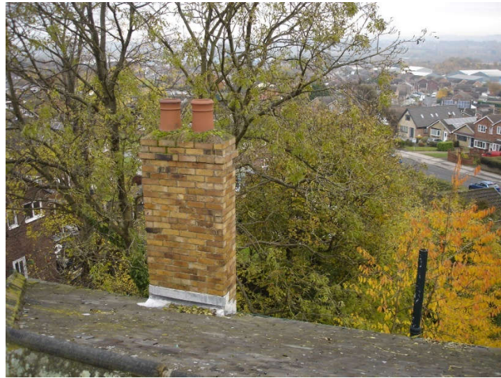
Fig 15. The rear of two brick-built chimney stacks on the east elevation.
