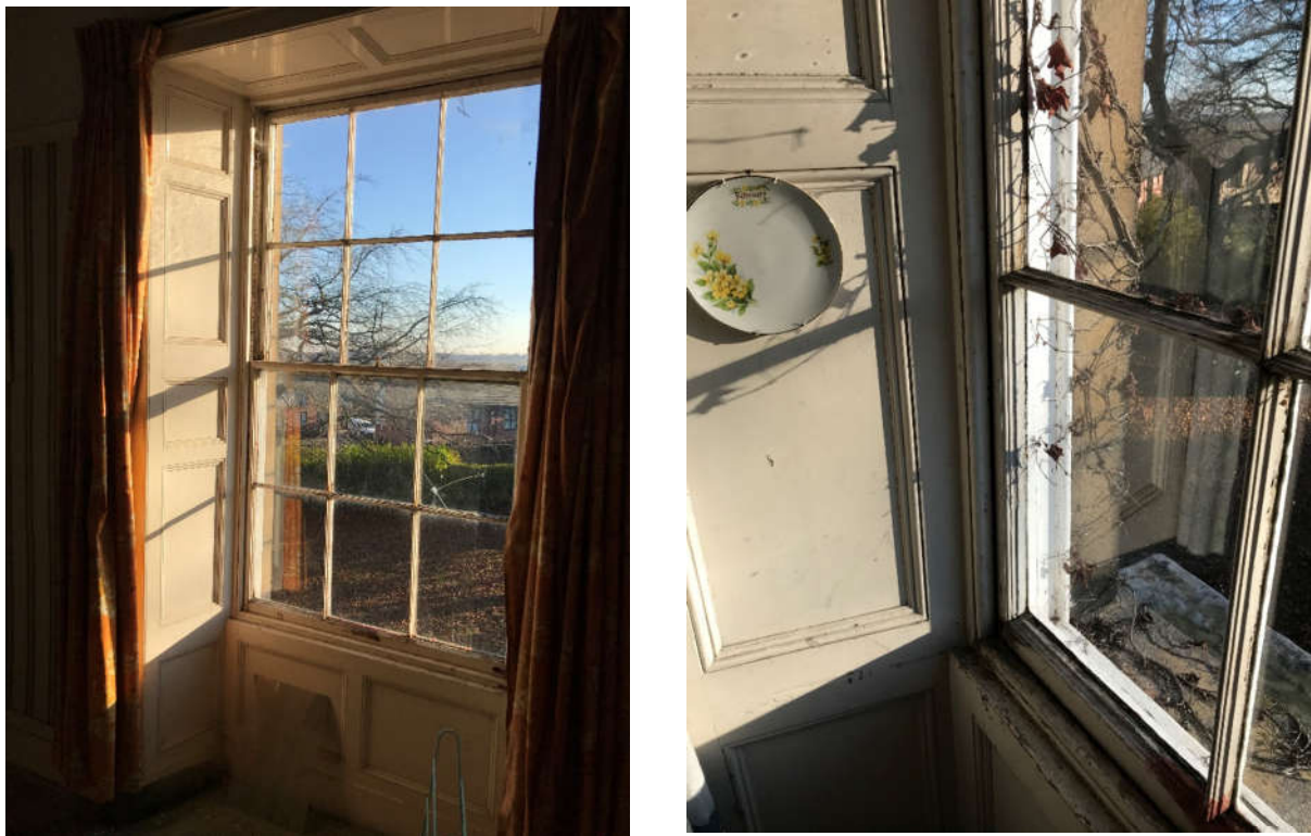
Fig 22. Typical interior views of sash windows to south elevation.
