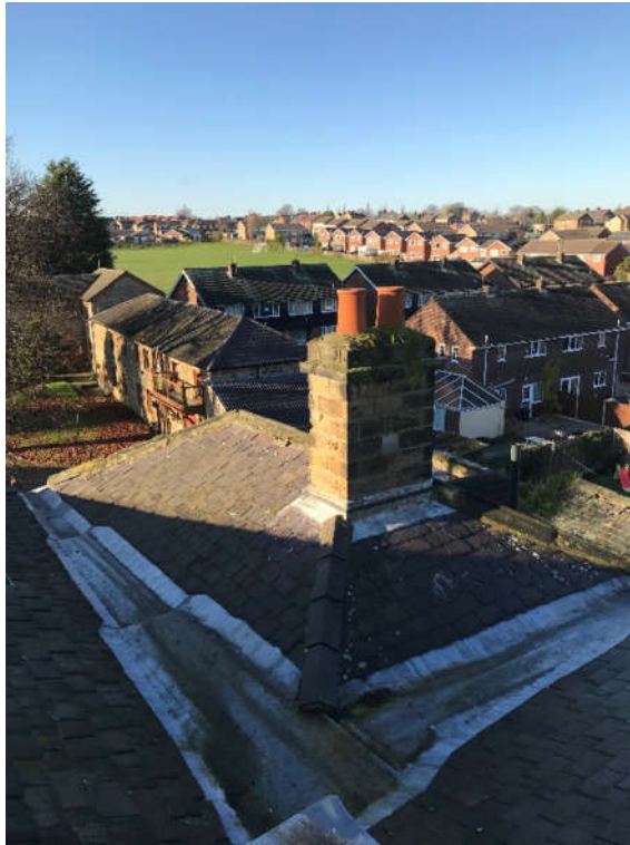
Fig 24. Chimney stack on rear hipped roof above Bed 6.
