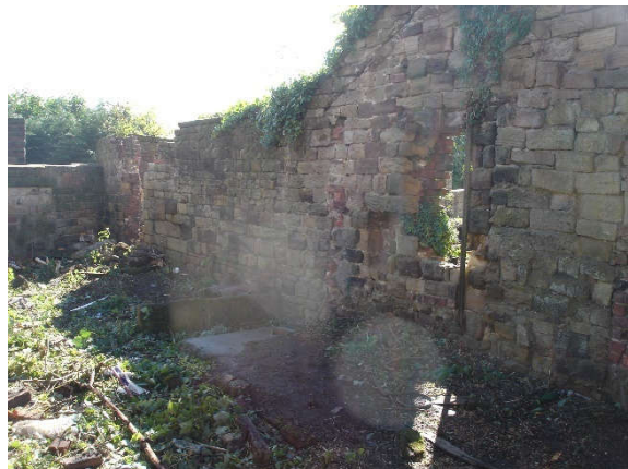
Fig 12. Garden wall north side.
