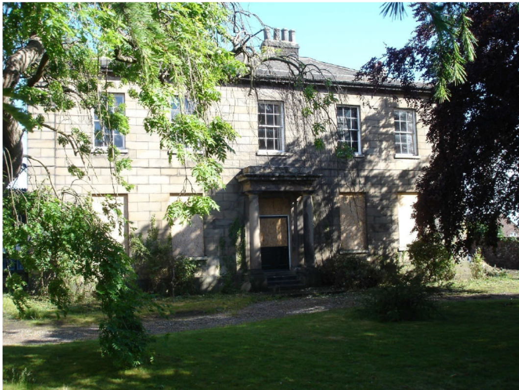
Fig 01. Front [South] Elevation of Osborne House
