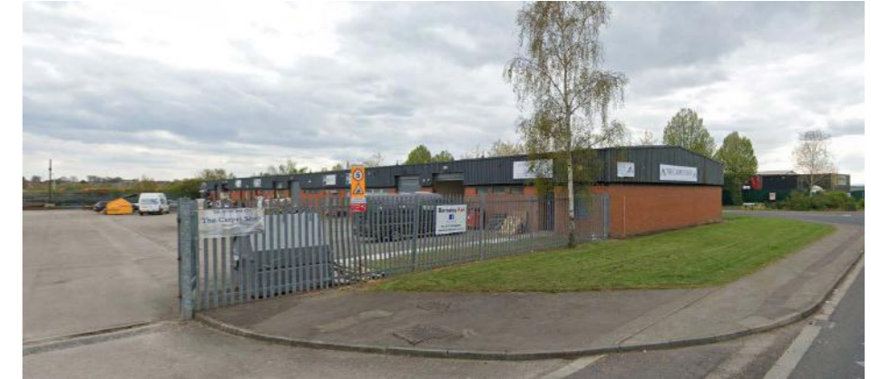
Photograph 08 - Multiple Occupied Units
