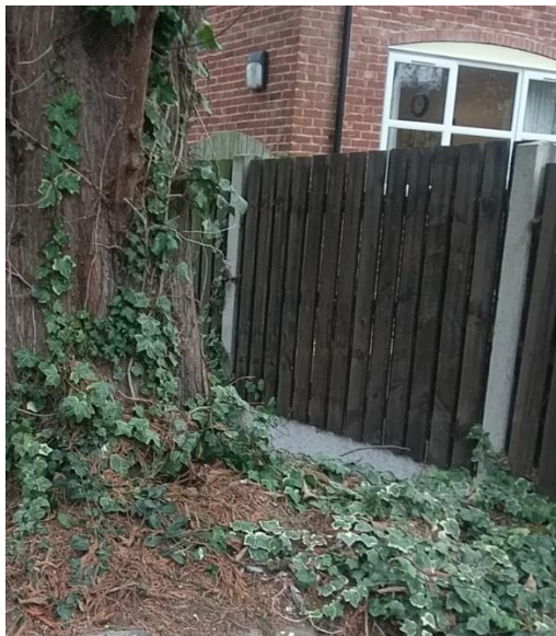
Fig. 5 – Existing vertical boarded fence with concrete posts and base rail.
