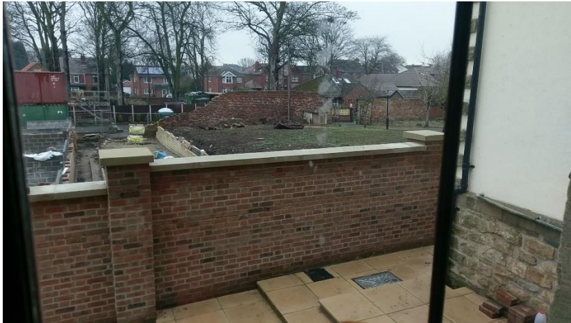
Fig. 4 - New brick wall with piers and PC copings to north-west boundary.
