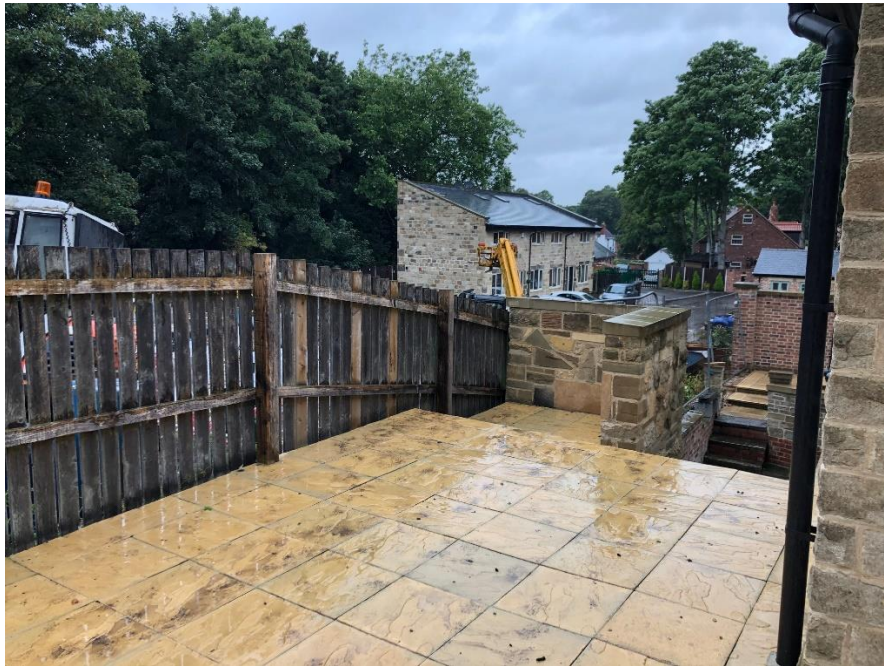
Fig. 3 – Existing Timber Fence to upper external level – proposed to be replaced
