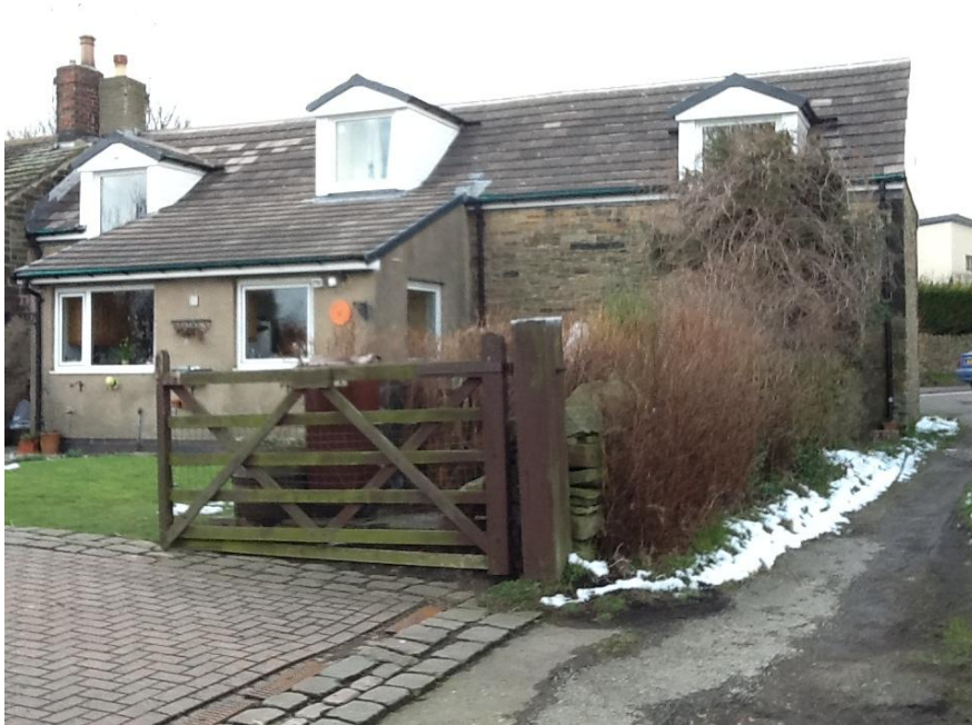
view of rear elevation
