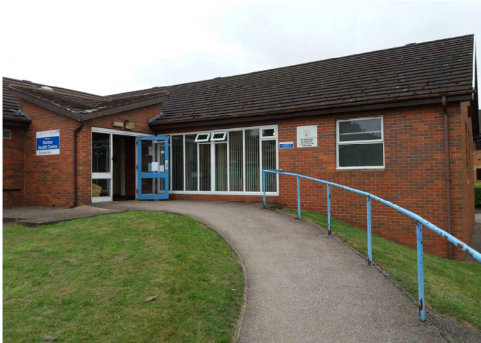
Photo showing closer view of sloping entrance
