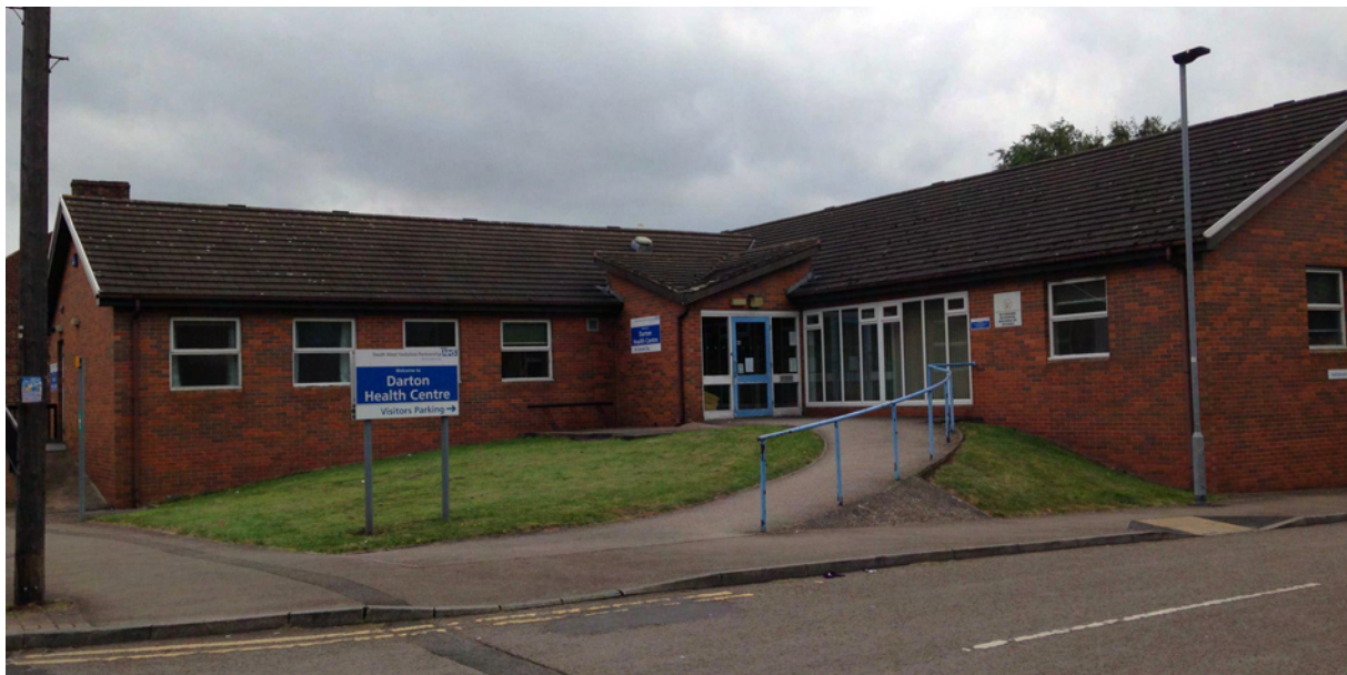
Photo of the existing entrance access slope and grassed areas
