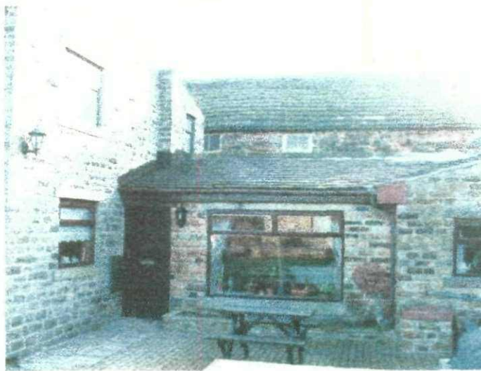
Photo of Front Elevation of Existing Building:
