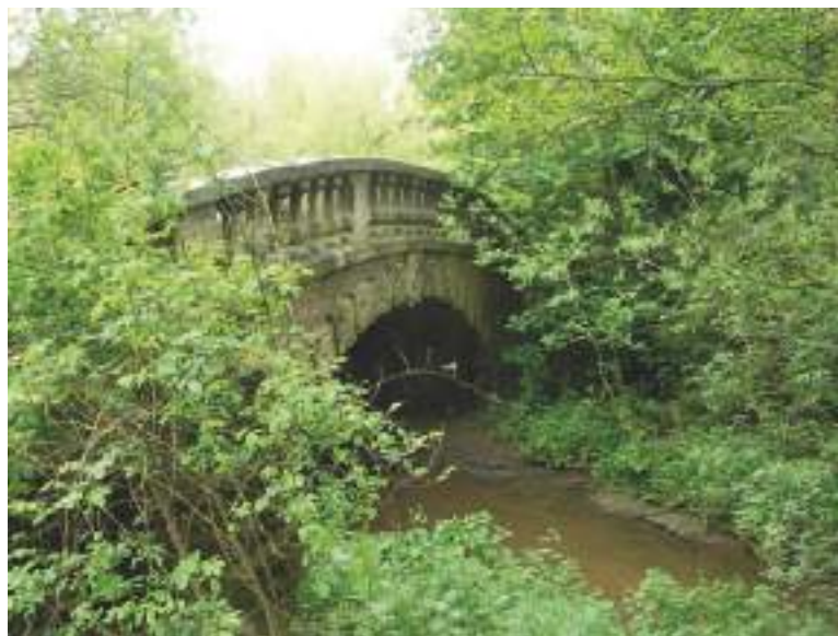
Figure 74. The bridge seen from upstream, 2016.
