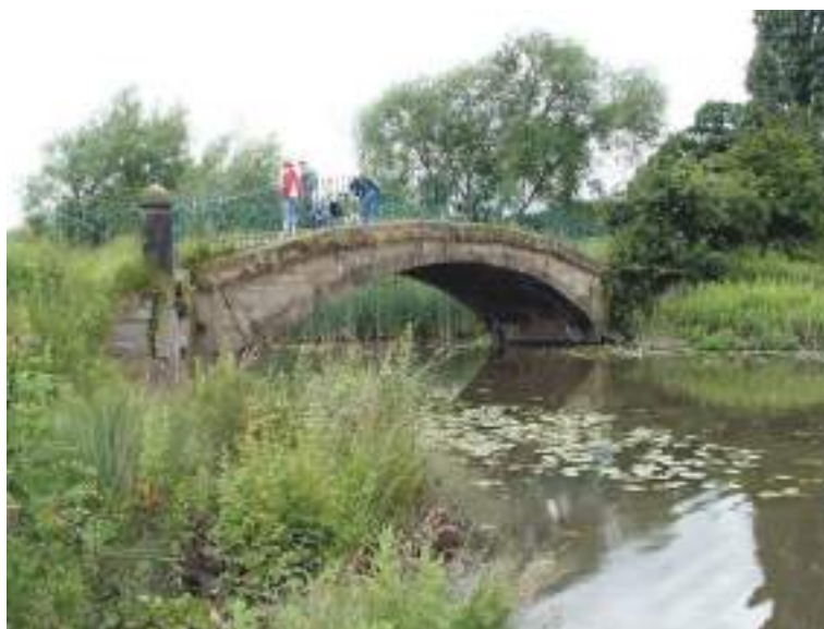
Figure 76. The “Palladian Bridge”
