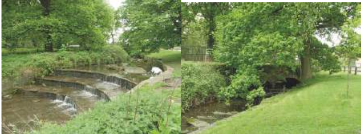
Figure 43 Overflow channel and waterfall, 2016
