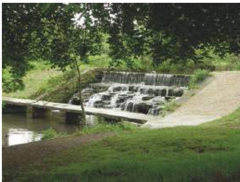
Figure 52. First cascade and footbridge.
