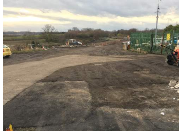
Western end of site showing recently re-graded landscaping to west
