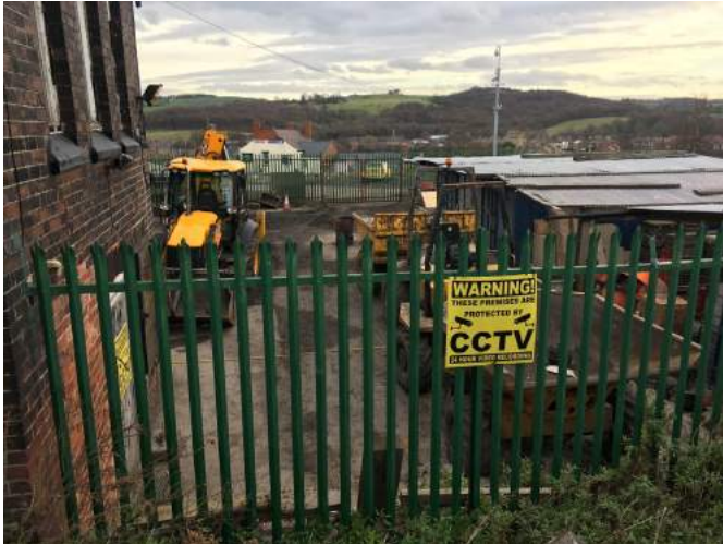
Compound area in North west of site adjacent to existing building
