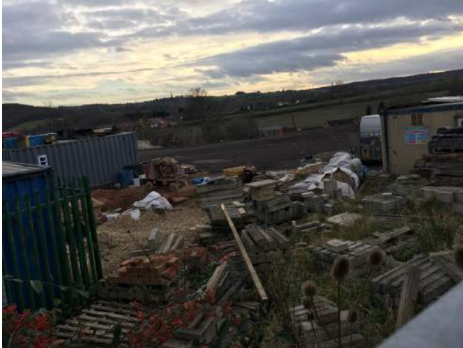
Building materials stored in north of the site
