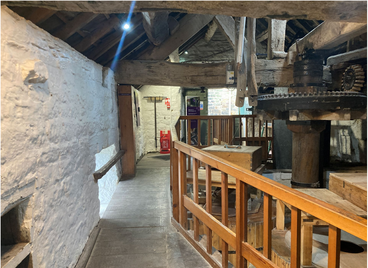
Plate 3: First floor of the 17 th century portion showing the existing 20 th century access ramp.
