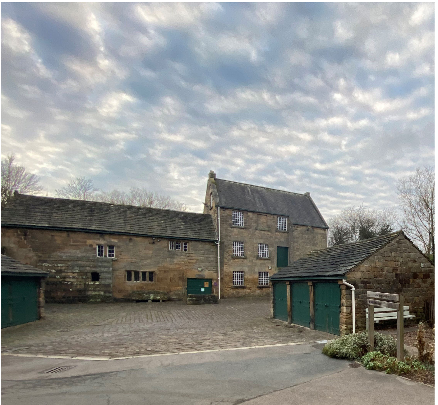
First Floor Access Ramp
