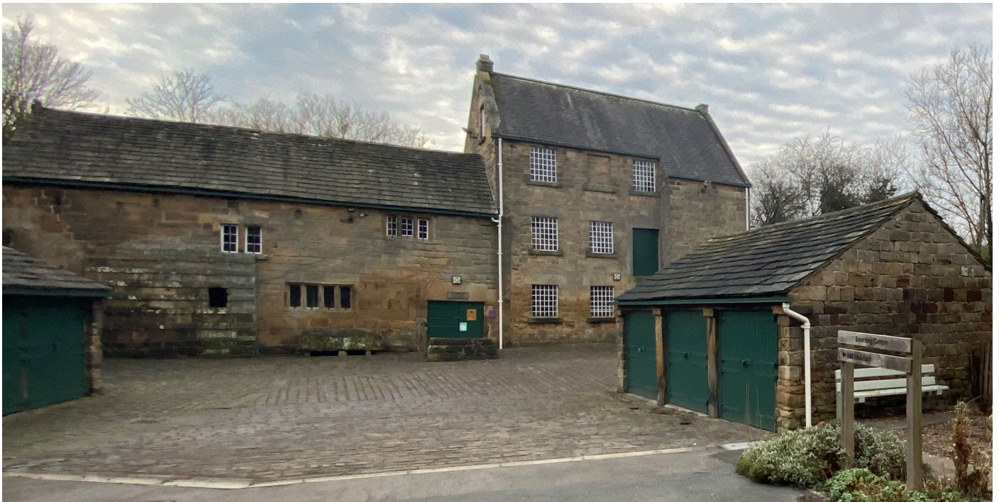
Plate 2: Worsbrough watermill with the 17 th century segment on the left and the 19 th century extension on the right.
