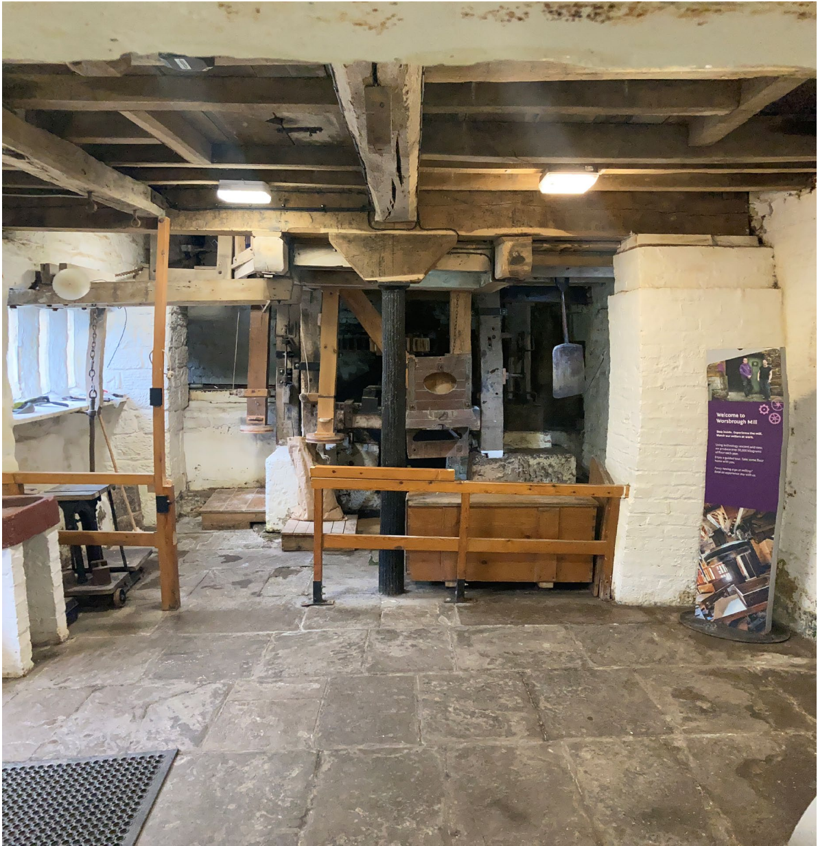
Plate 7: Ground floor area beneath the new ramp and mill machinery.
