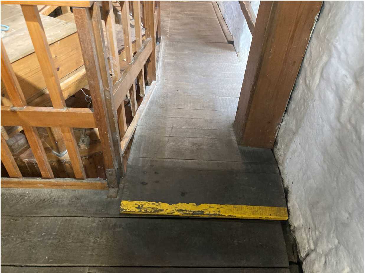
Plate 5: Step at the top of the 20 th century ramp.
