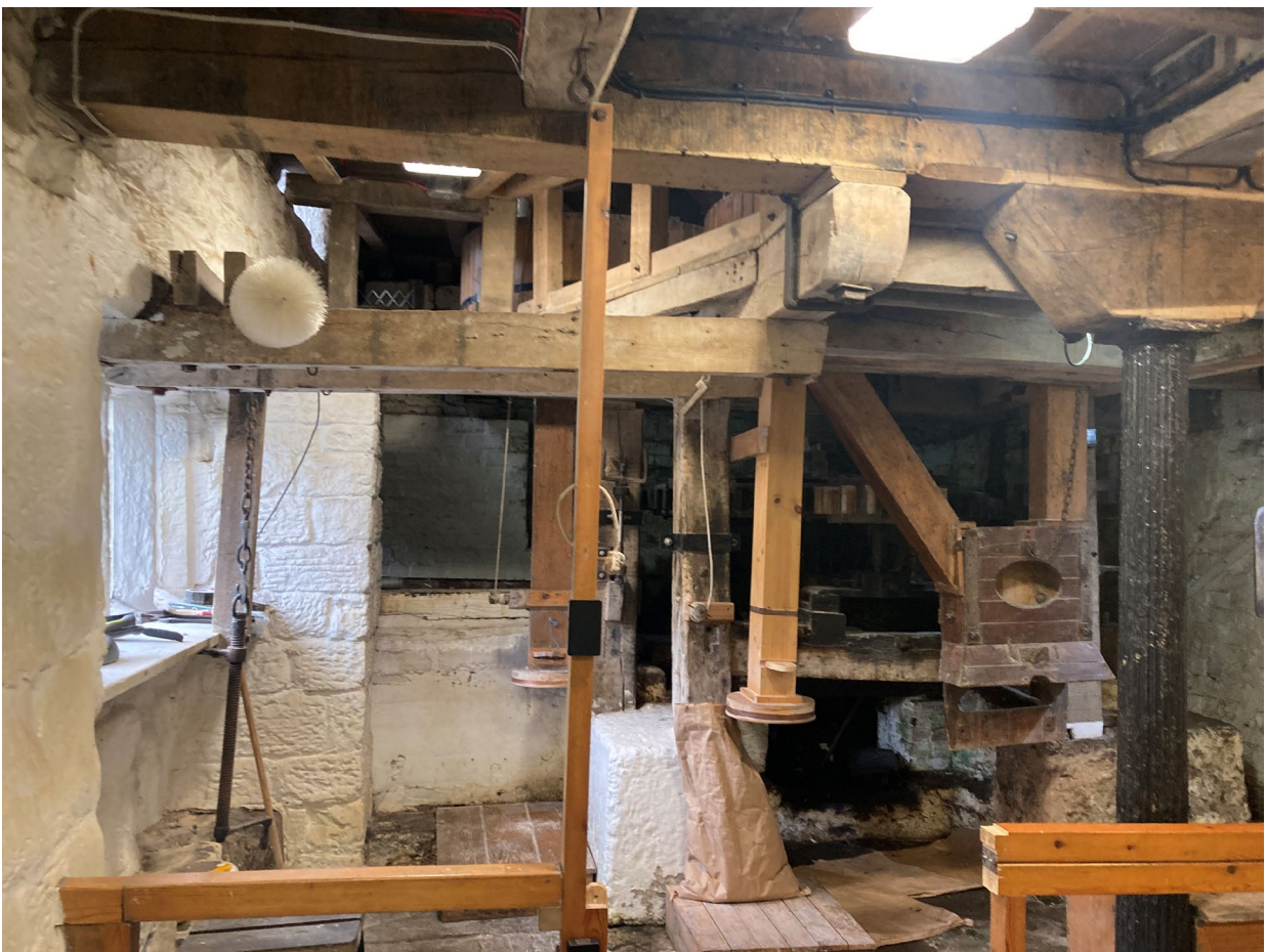
Plate 6: Ground floor ceiling showing location of floor to be infilled.
