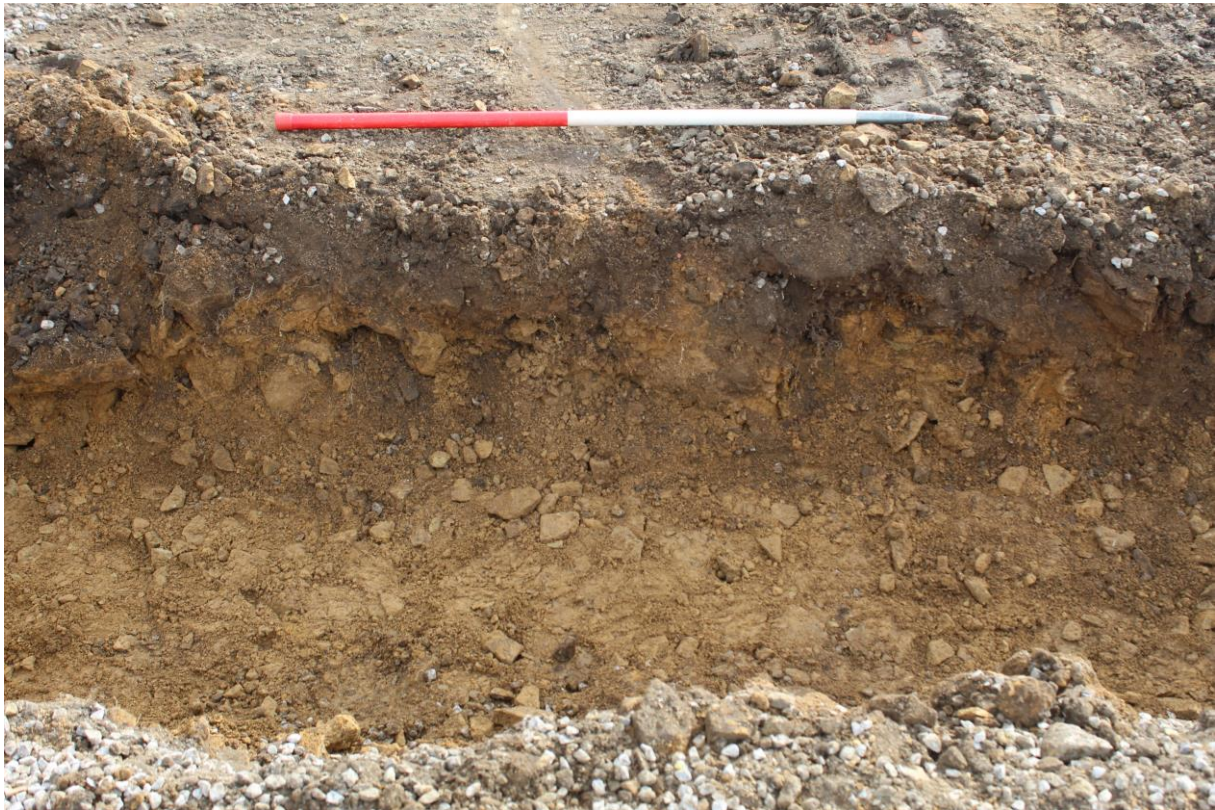
Plate 3: Section of Footing, facing East.
