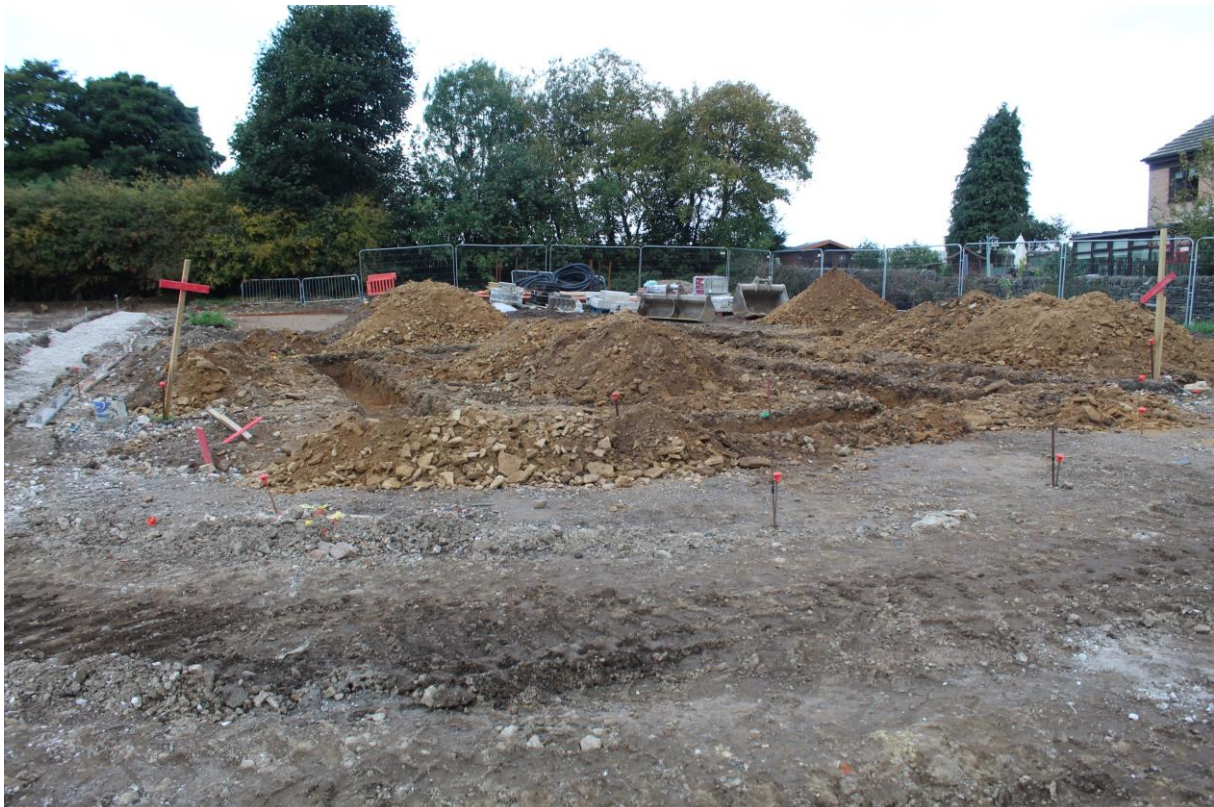
Plate 2: General Shot of Footings, facing West.
