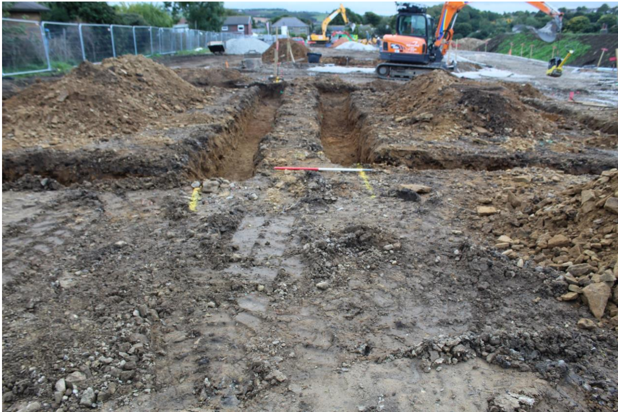
Plate 1: General Shot of Footings, facing East.
