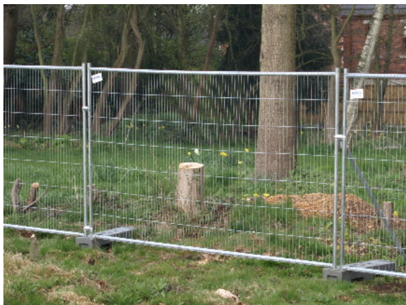
Tree protection fencing.
