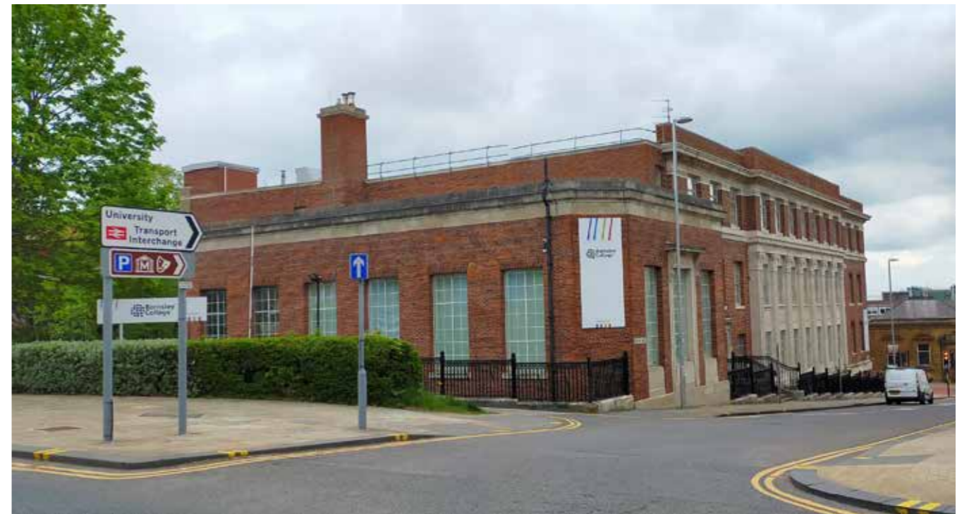
Photograph of West Elevation from St Mary's Place
