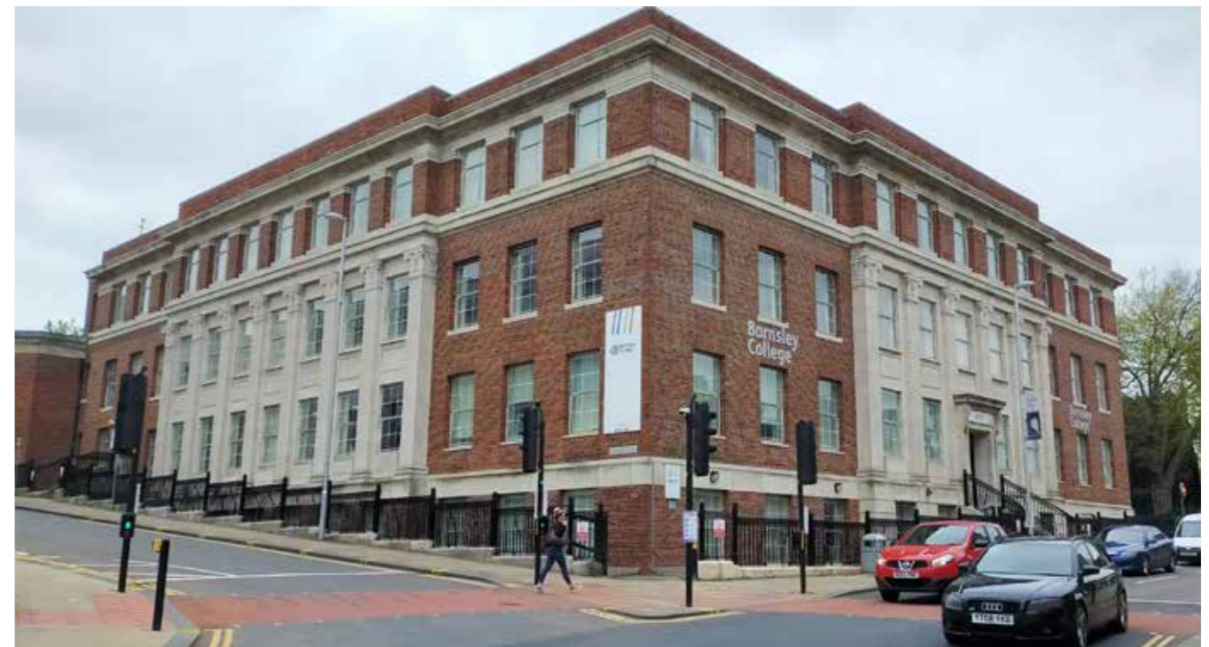
Photograph of Barnsley College Church Street Campus from Church Street
