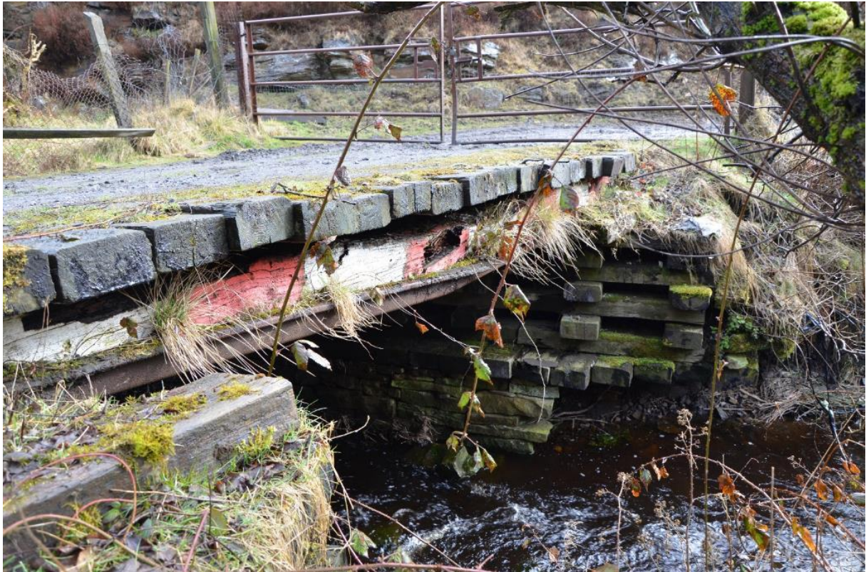
Plate 11: RSK 088 stone bridge abutments beneath modern timber bridge supports
