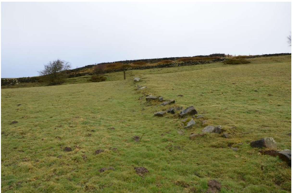
Plate 10: RSK 087 collapsed drystone wall
