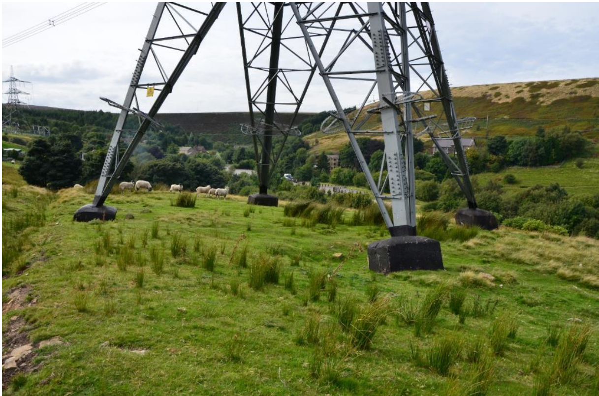
Plate 1: RSK 007 Remnant dry-stone wall boundary adjacent to Pylon 4ZO162
