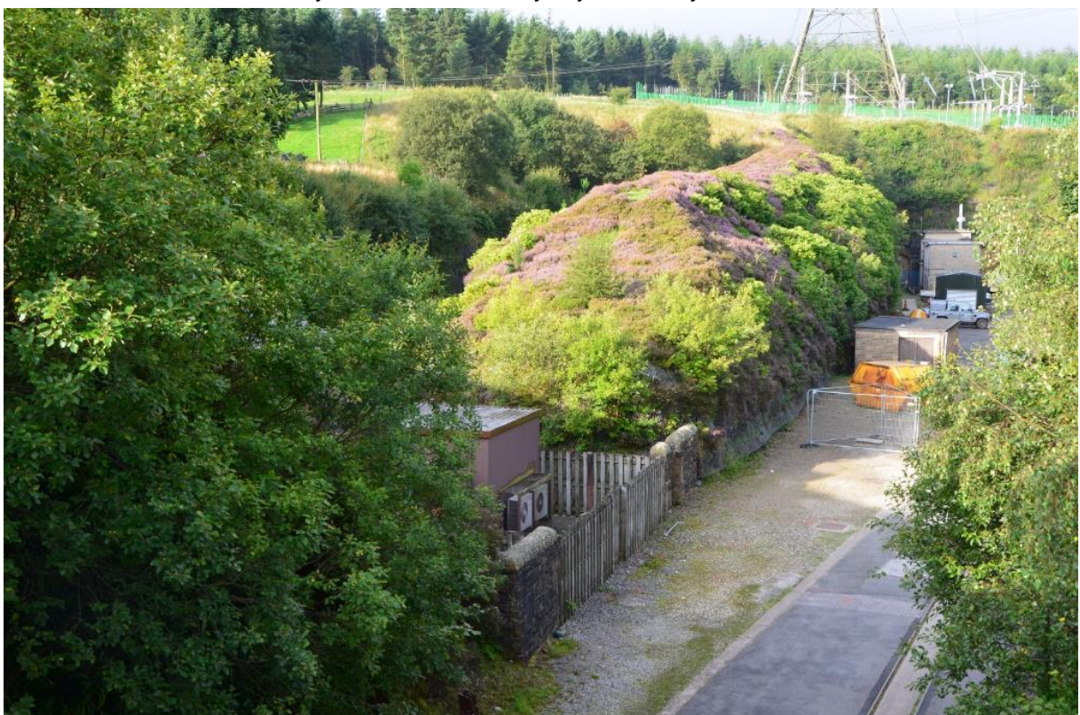
Plate 2: RSK 016 rocky embankment within Woodhead Tunnel Portal (NB: Mitigation no longer required in this location)
