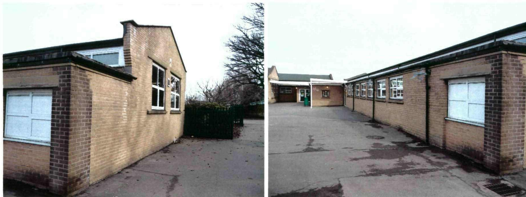
Photographs showing the existing West and North facing elevations
