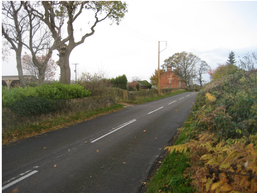
2. Existing access looking south west
