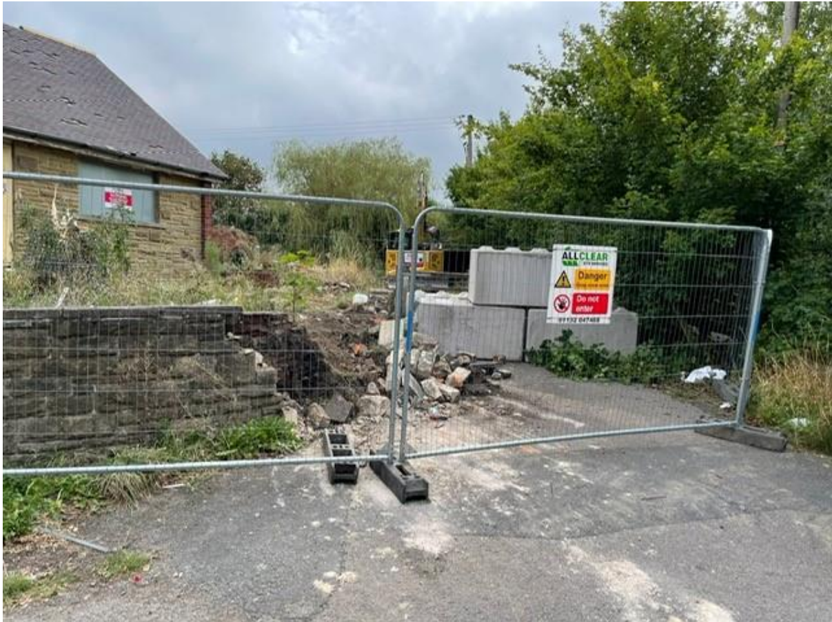
Appendix 3: Photos showing start made on site
