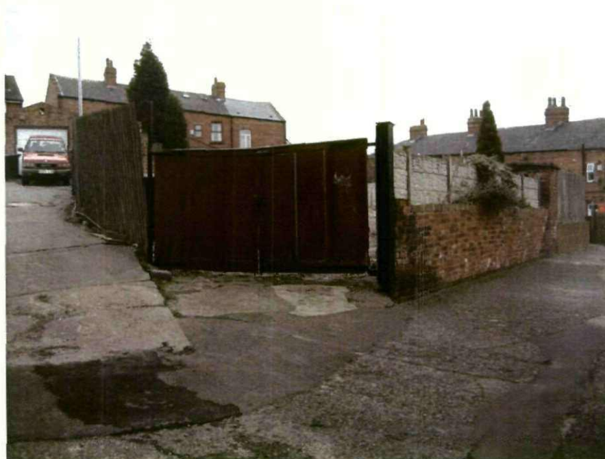
2. Existing access to former wood yard at North Eastern corner of the site
