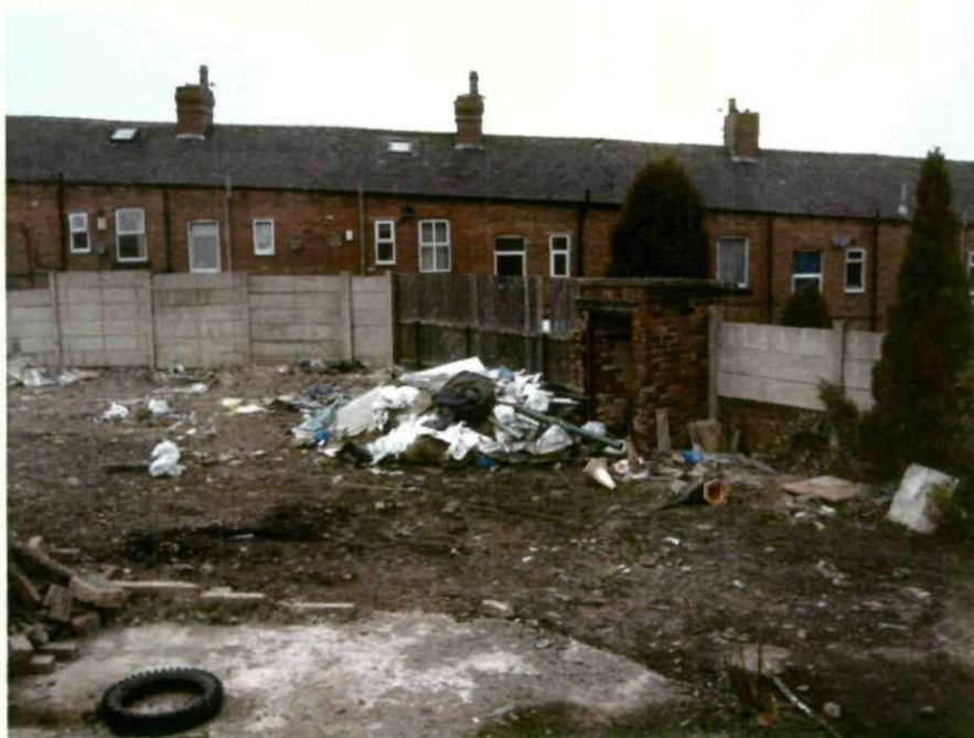
8. Internal view of West and Northern boundary with terraced housing to rear
