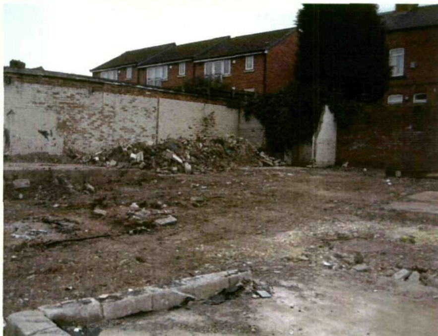
5. View into South Eastern corner of the site
