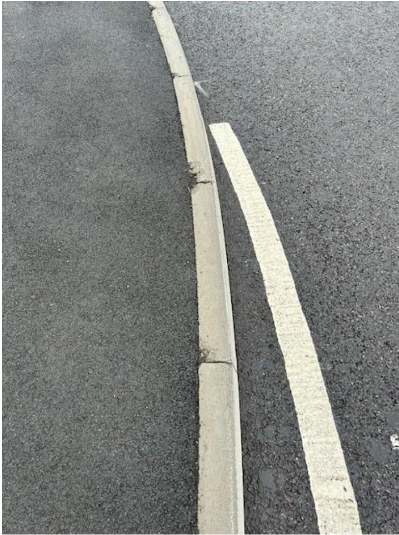
Image 8 – Damaged kerbs
