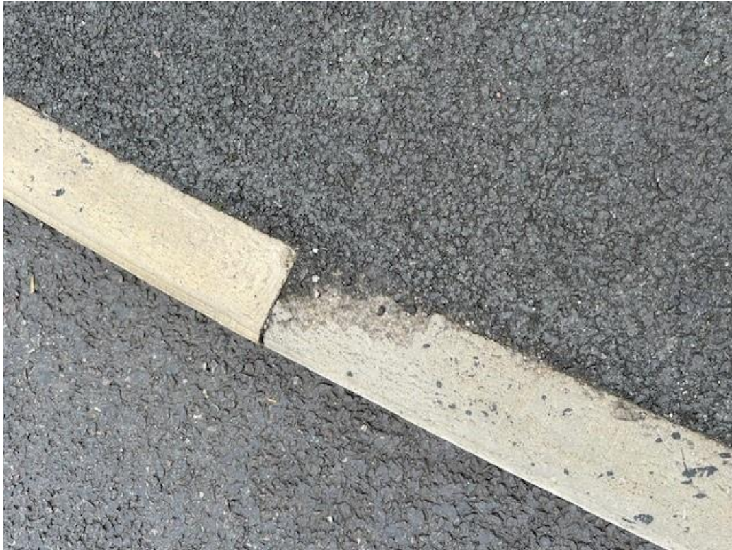
Image 9 – Damaged kerb
