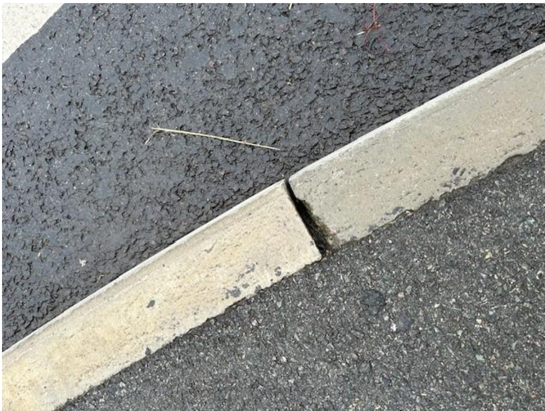
Image 10 – Damaged kerb
