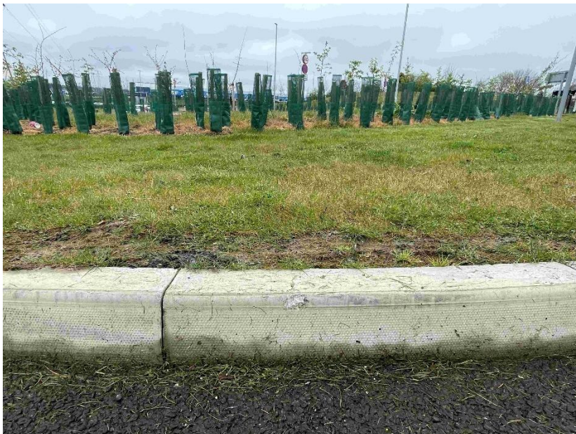
Image 17 – Chipped kerb
