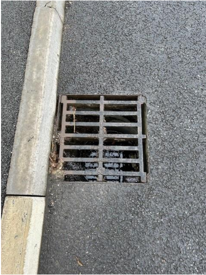
Gully 1 to Sheffield Road (Site access road)
