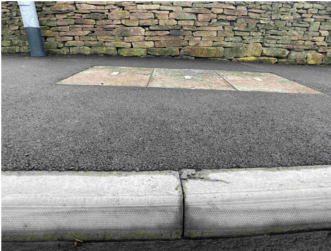
Image 4 – Damaged Kerb
