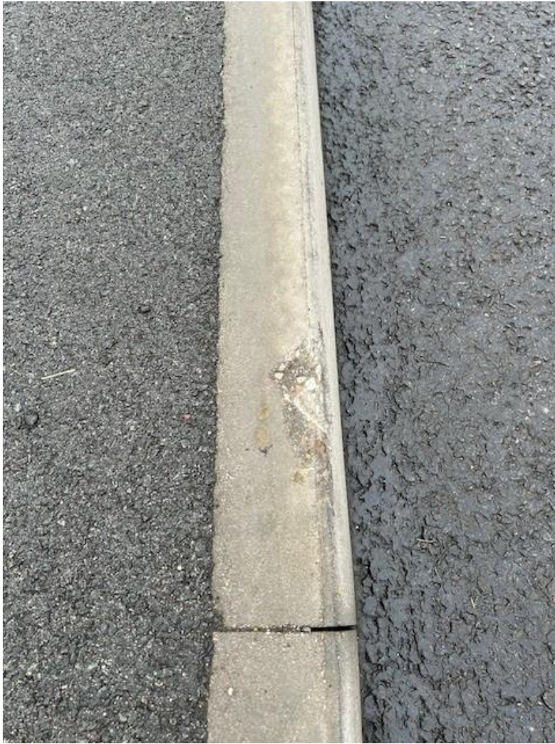
Image 12 – Chipped kerb
