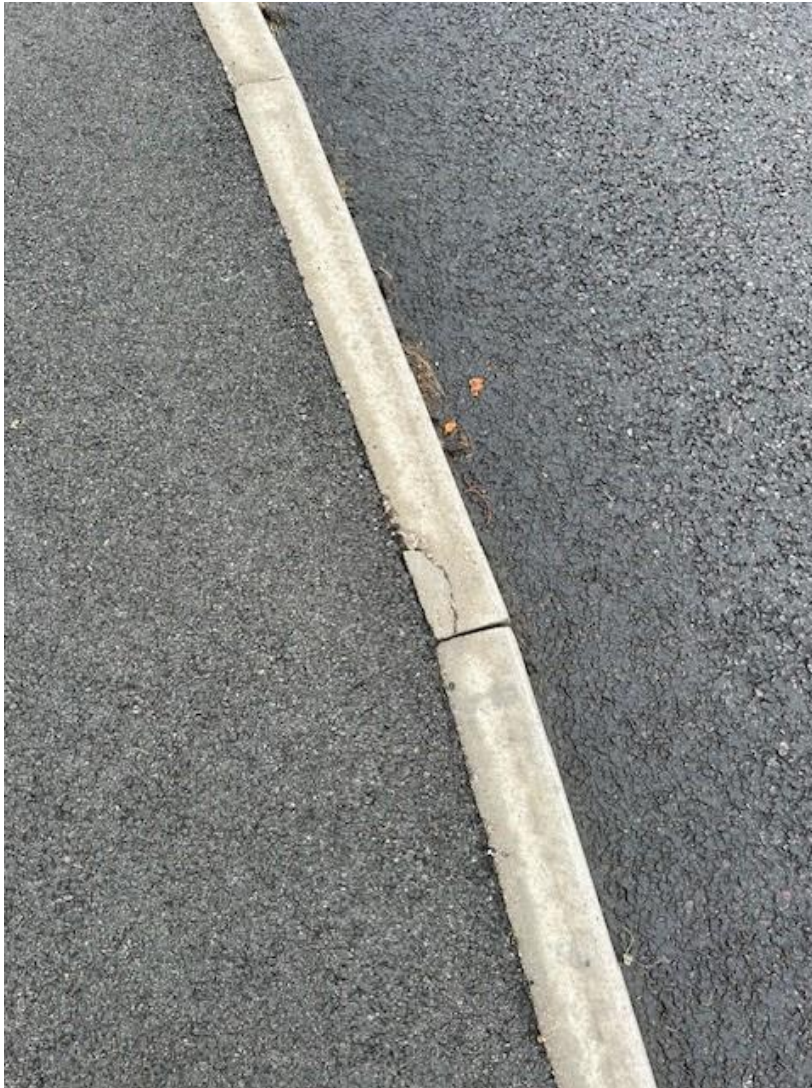
Image 11 – Cracked kerb
