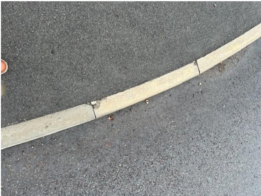
Image 5 – Damaged kerb
