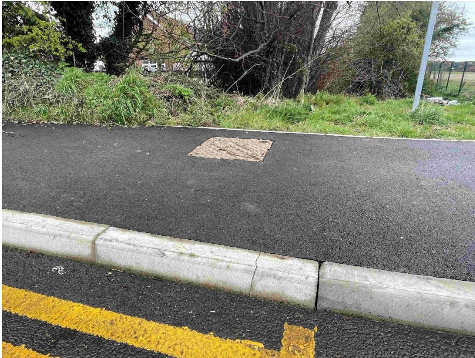
Image 2 – Cracked Kerb
