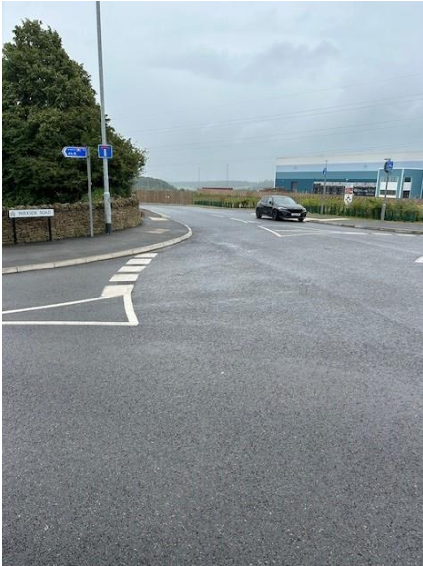
Roundabout looking South
