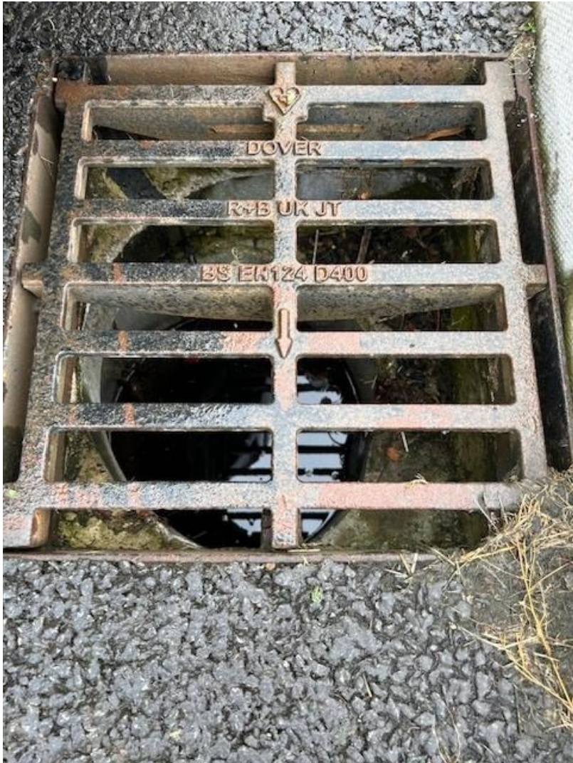
Gully 2 to Sheffield Road (Site access road)
