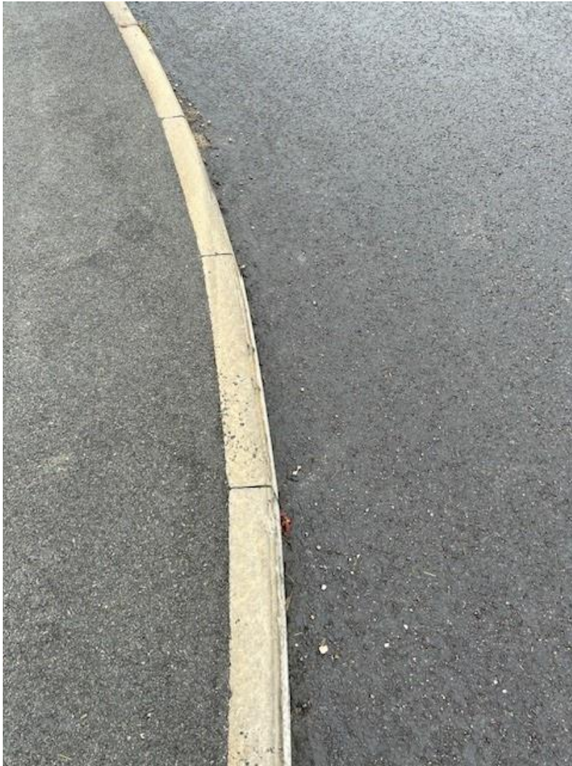
Image 13 – Chipped kerb
