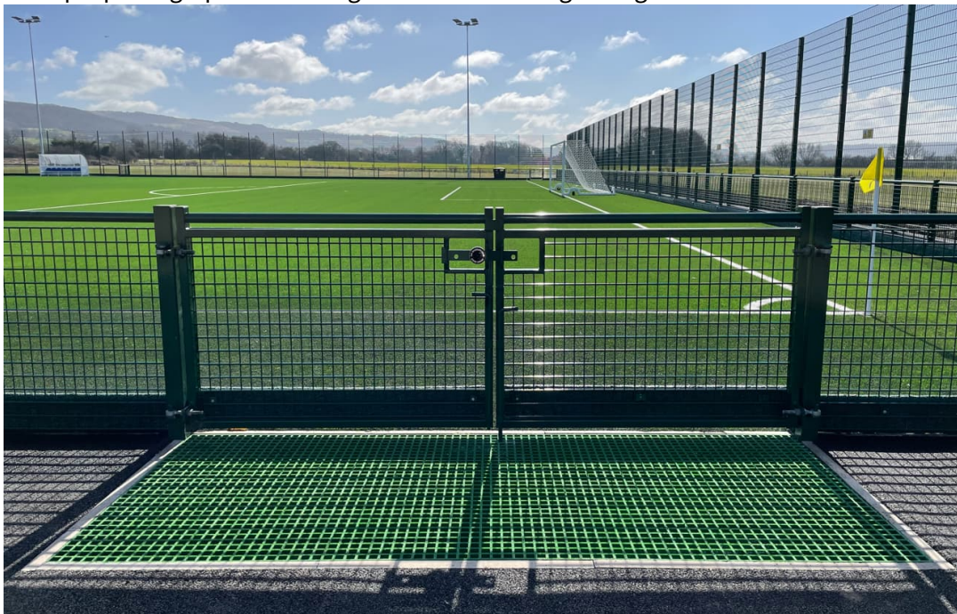
Example photograph of double gate with in-fill mitigation grate:
