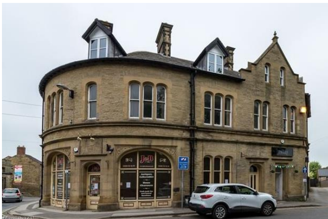
Figure 4 – Midland Bank and Bank Chambers, St Mary's Street is a grade II listed building with an entry number of 1286793.
