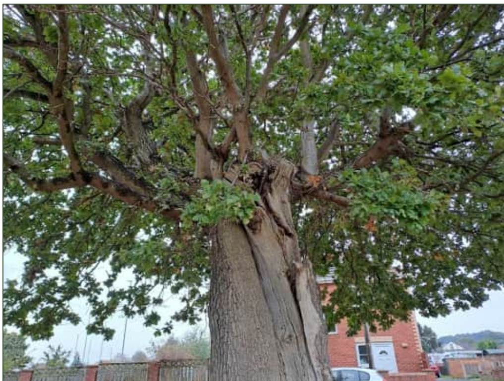
Plate 3-10: Large cracks and fissures visible in the oak tree situated on the eastern boundary of the Site. This tree is to be retained as part of the proposed development.
