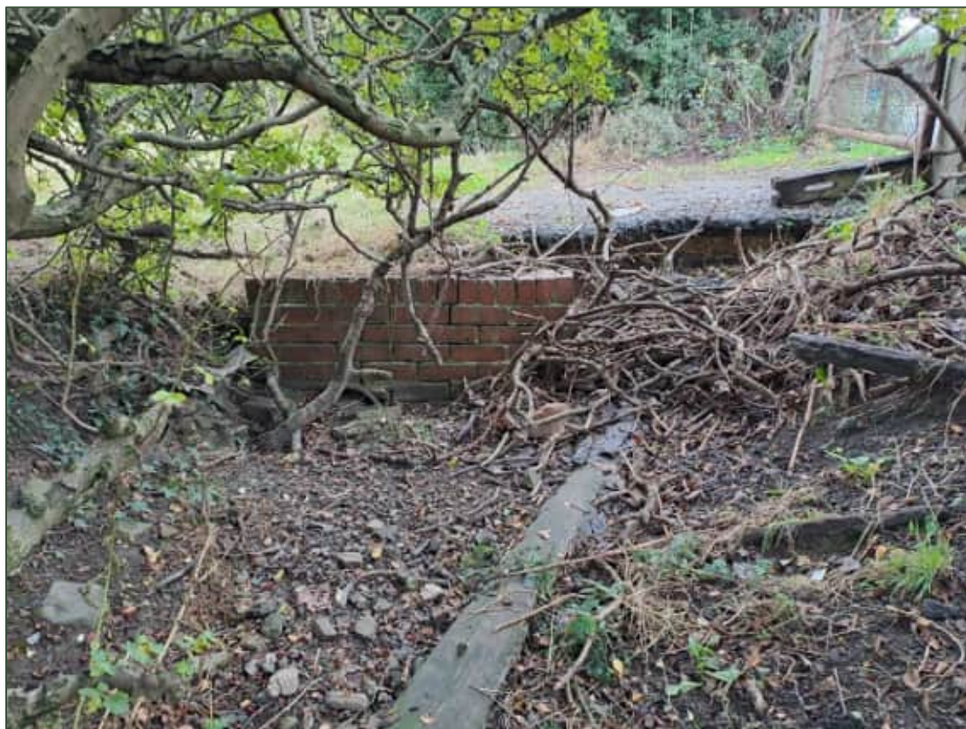
Plate 3-9: The culvert present in the northern ditch.
