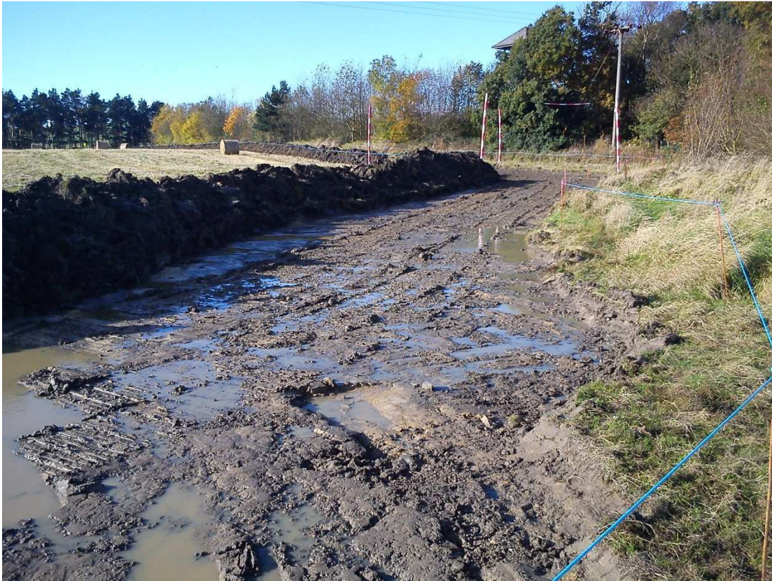
Photo 7: Existing utilities development on western boundary of the turbine field
