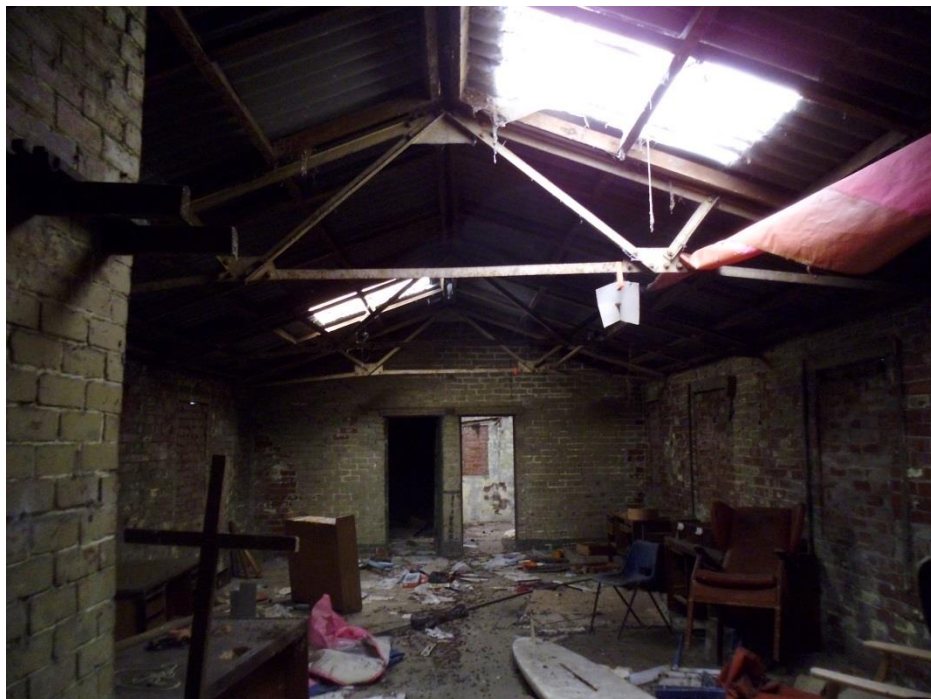
Plate 2 Inside of building showing steel frame supporting asbestos roof
