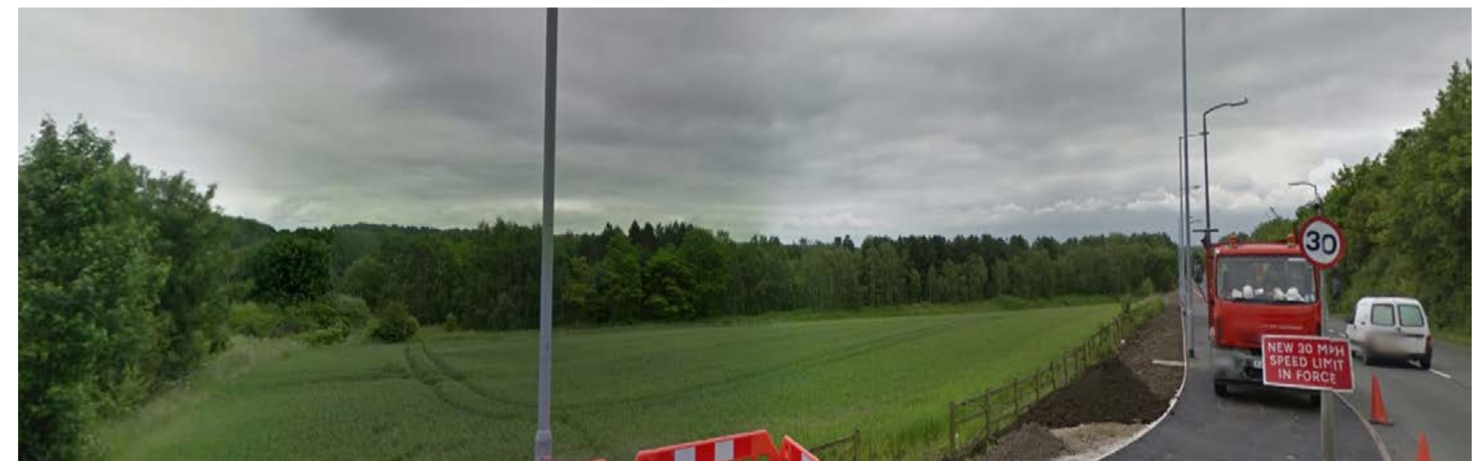
View of the North of the site [from Mitchells Way]
