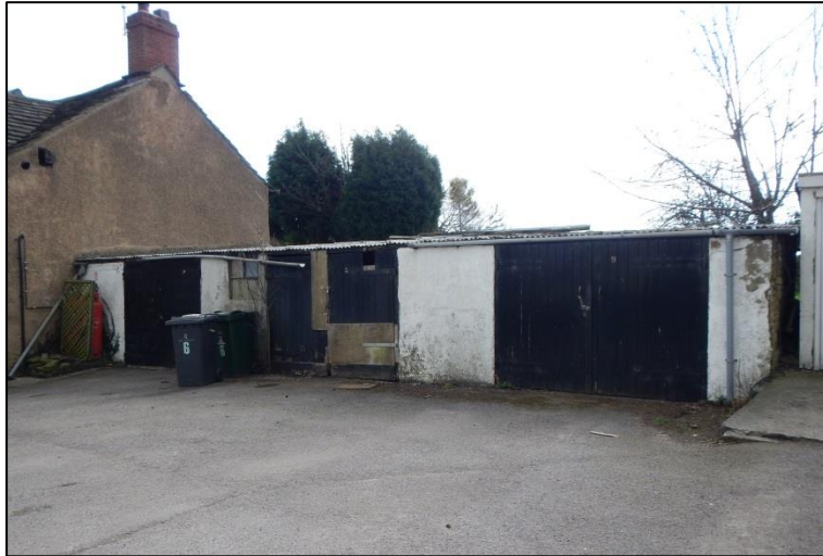
Figure 1: North facing aspect of the garage building
