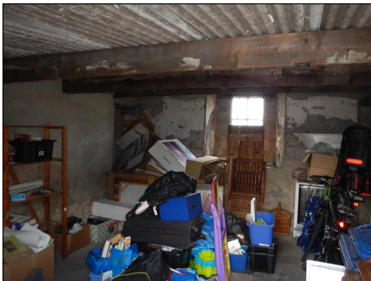
Figure 2: Internal view of a garage compartment
