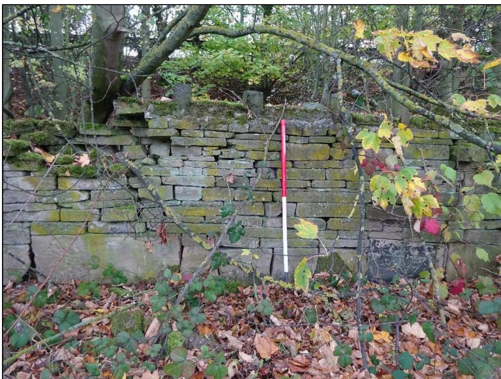
Plate 5: Wall to Higham Lane along north-western boundary of the Site
